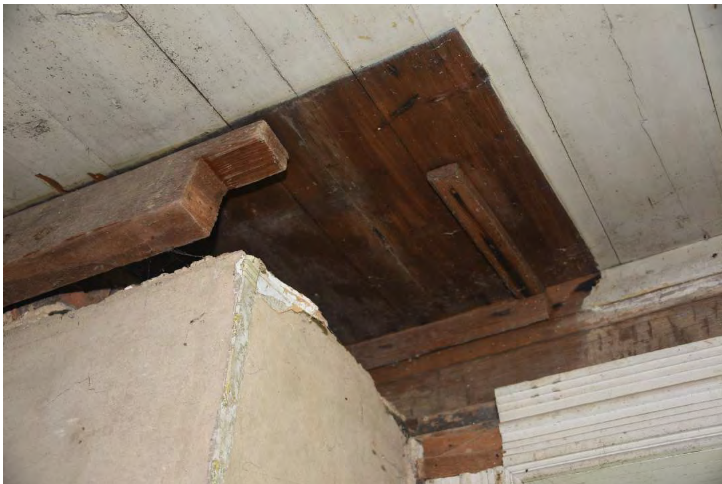
MD_FrederickCounty_Beatty-Cramer_0011.tif East room, ghost of original cabinetry at chimney.
