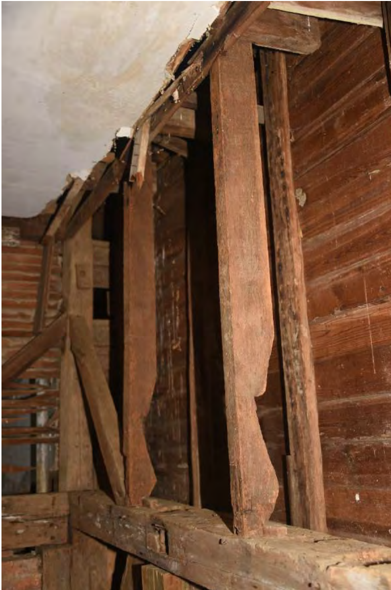
MD_FrederickCounty_Beatty-Cramer_0028.tif Center chamber, north wall with rafters reused as studs.
