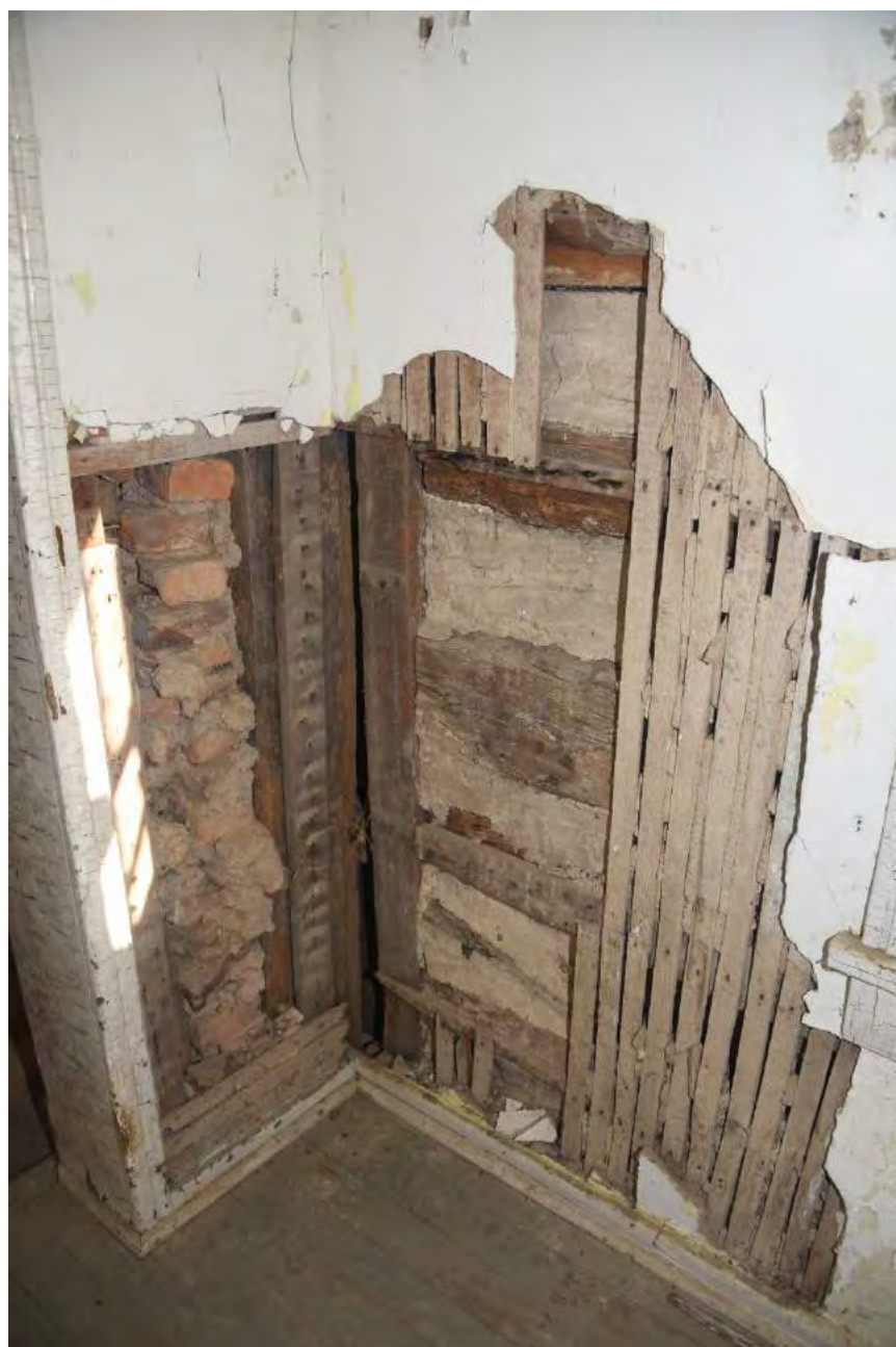
MD_FrederickCounty_Beatty-Cramer_0021.tif West room, southeast corner showing log wall with corner post.
