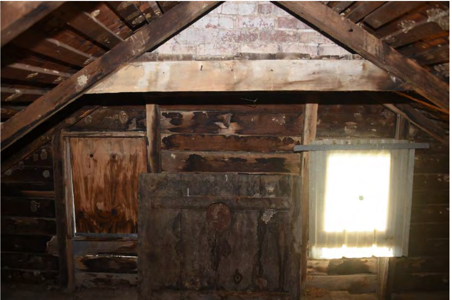
MD_FrederickCounty_Beatty-Cramer_0032.tif Attic, west elevation showing false chimney.
