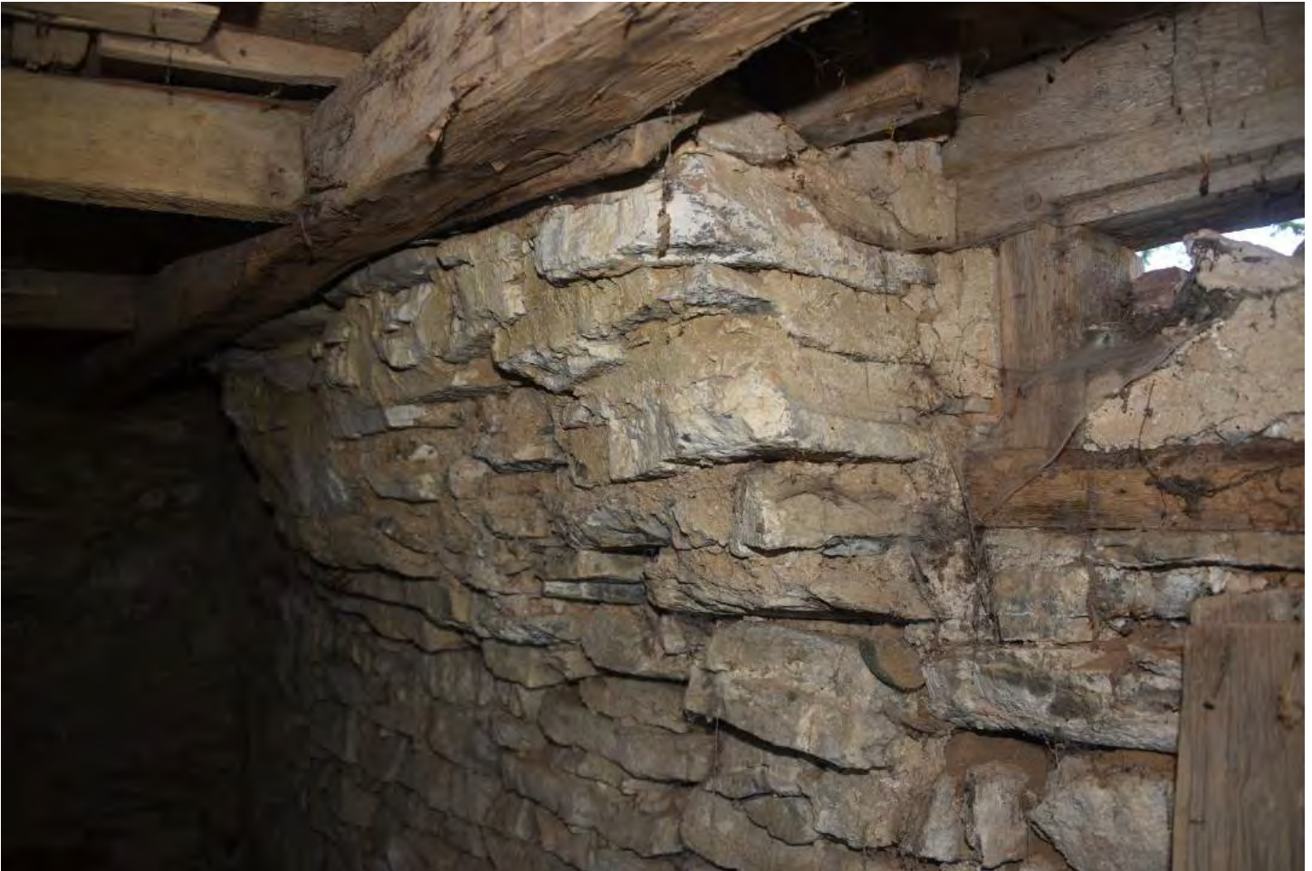
MD_FrederickCounty_Beatty-Cramer_0034.tif East basement, east wall corbel for fireplace.
