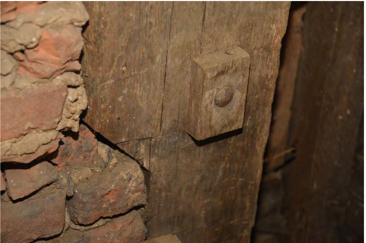
MD_FrederickCounty_Beatty-Cramer_0027.tif Center chamber, northwest corner post with jowl
