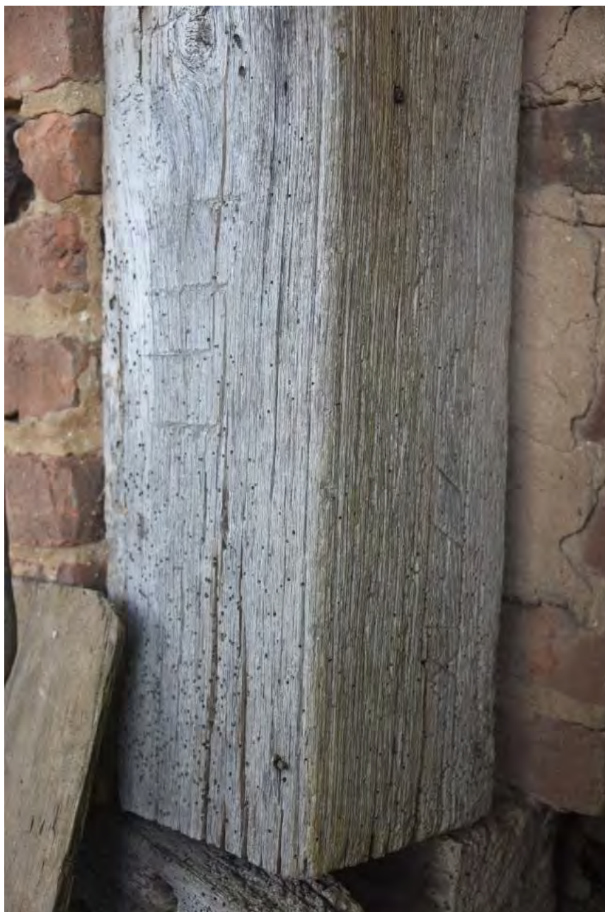
MD_FrederickCounty_Beatty-Cramer_0005.tif Northeast corner post with corner bead and marriage marks
