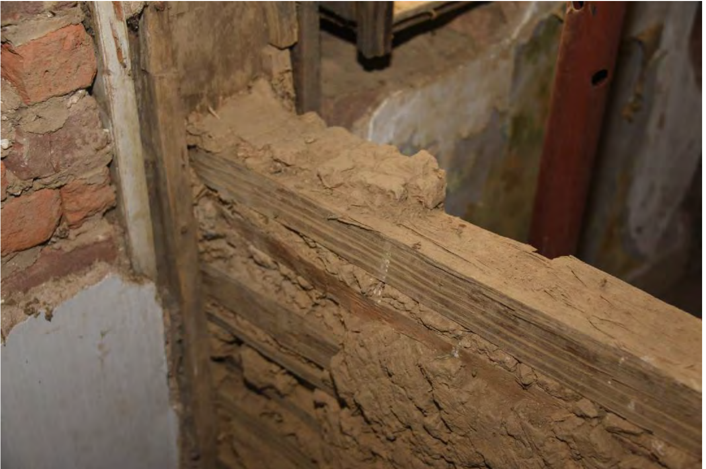
MD_FrederickCounty_Beatty-Cramer_0025.tif East chamber, southwest corner Dutch biscuit detail.
