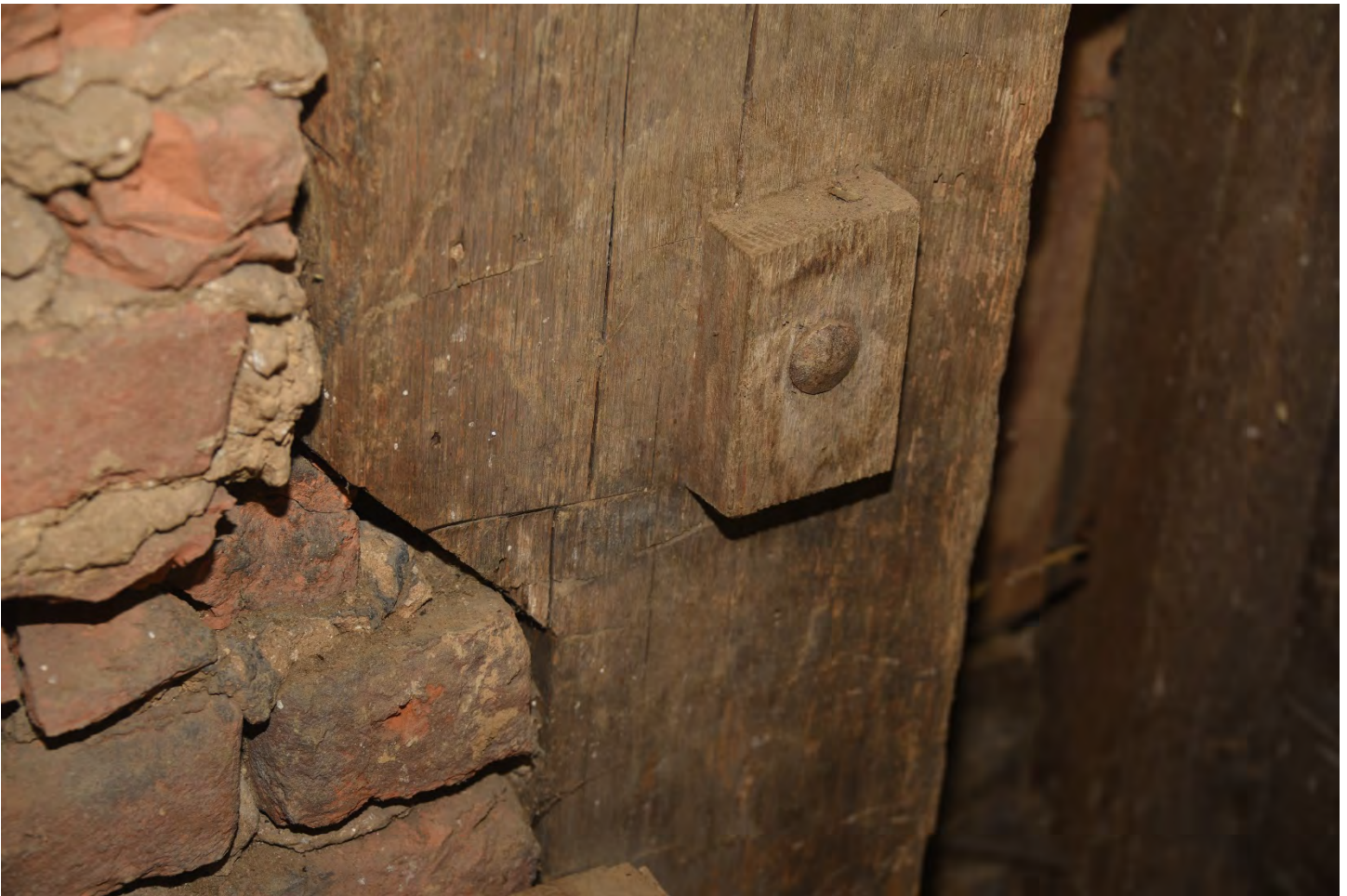
MD_FrederickCounty_Beatty-Kramer_0027.tif Center chamber, northwest corner post with jowl
