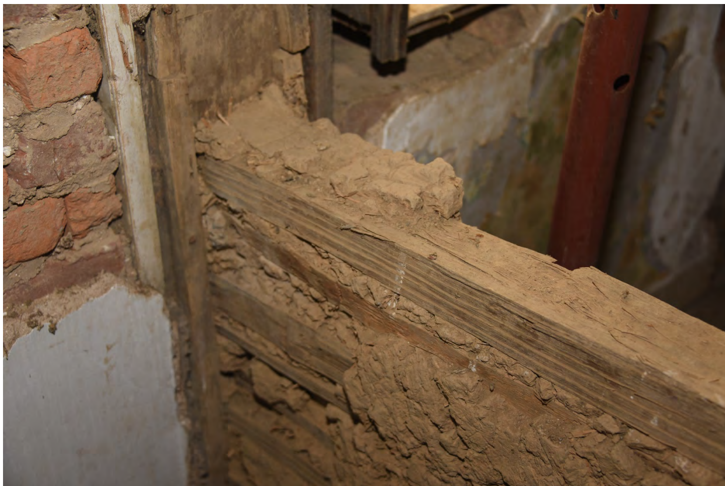
MD_FrederickCounty_Beatty-Kramer_0025.tif East chamber, southwest corner Dutch biscuit detail.
