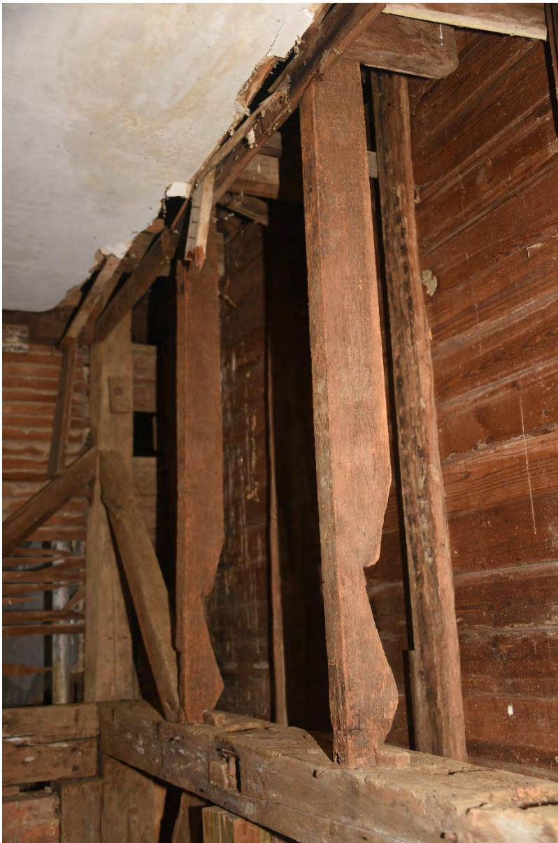
MD_FrederickCounty_Beatty-Kramer_0028.tif Center chamber, north wall with rafters reused as studs.
