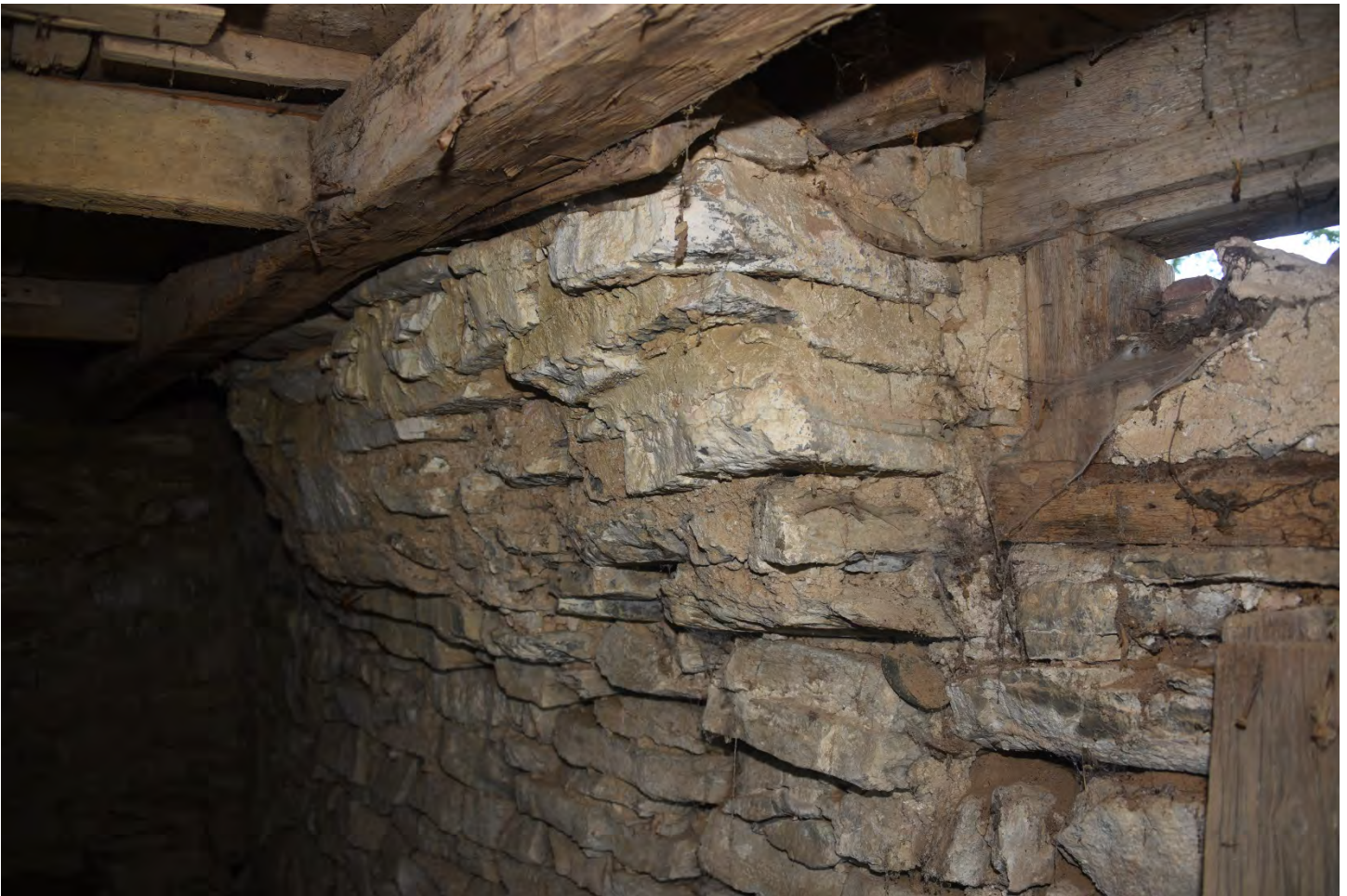
MD_FrederickCounty_Beatty-Kramer_0034.tif East basement, east wall corbel for fireplace.
