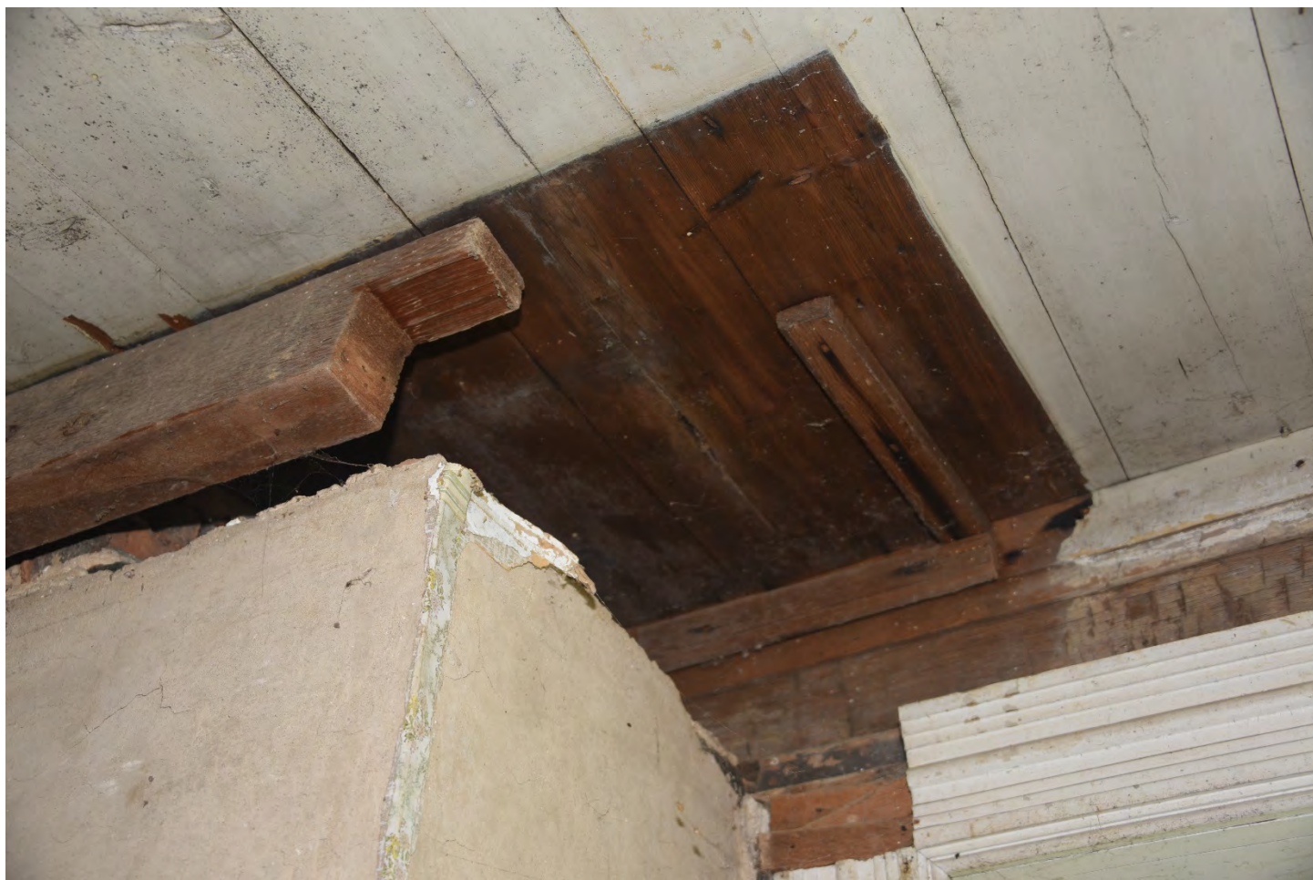
MD_FrederickCounty_Beatty-Kramer_0011.tif East room, ghost of original cabinetry at chimney.
