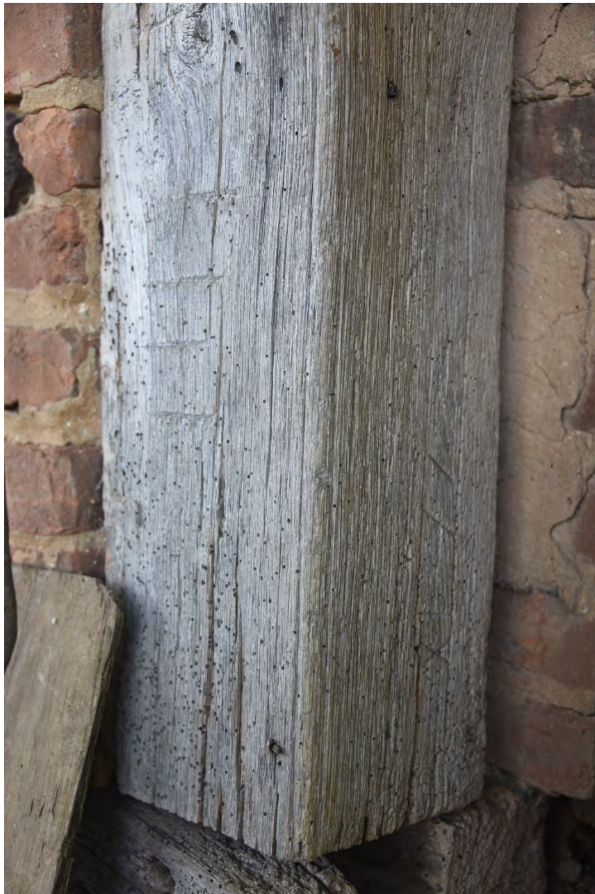
MD_FrederickCounty_Beatty-Kramer_0005.tif Northeast corner post with corner bead and marriage marks
