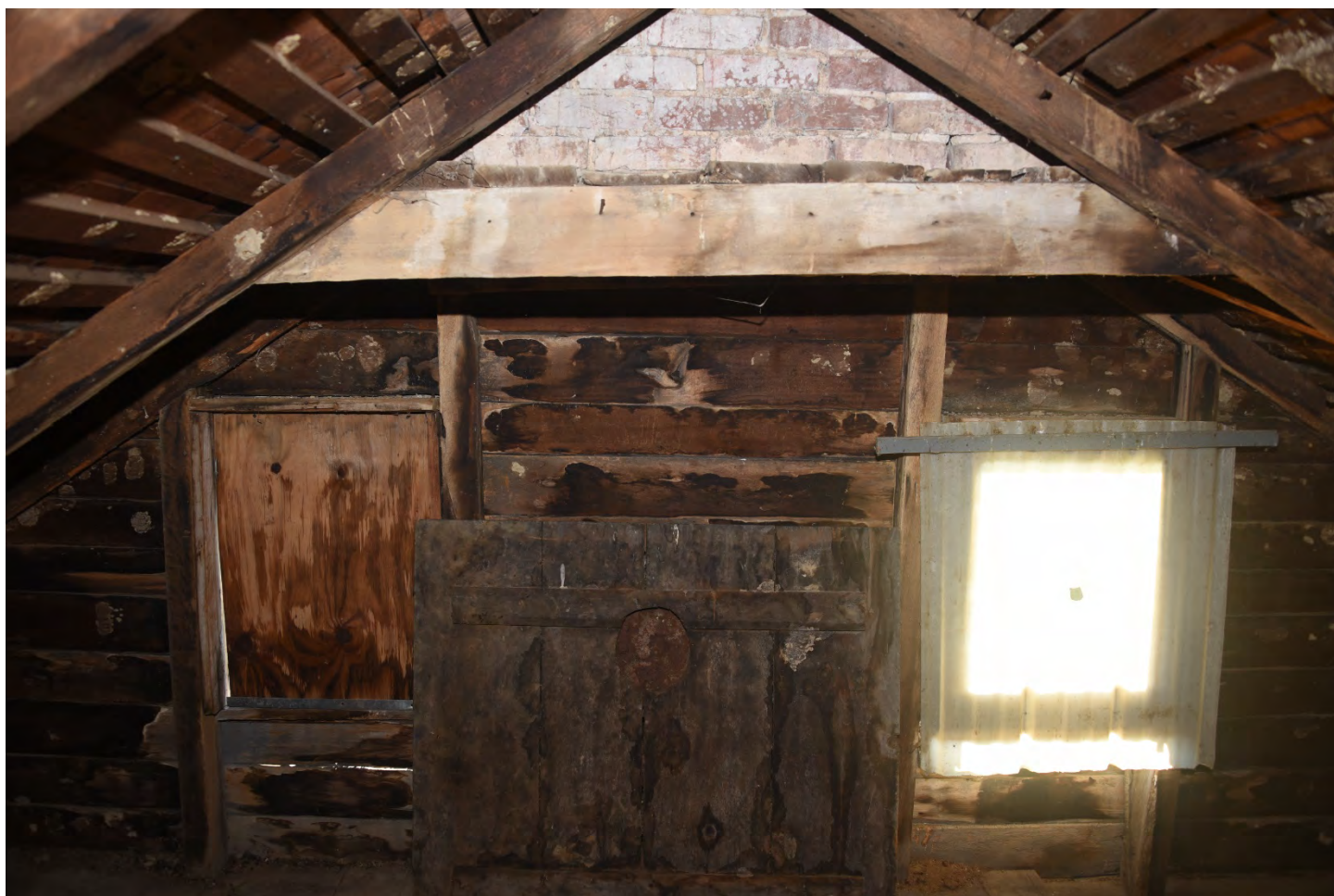
MD_FrederickCounty_Beatty-Kramer_0032.tif Attic, west elevation showing false chimney.
