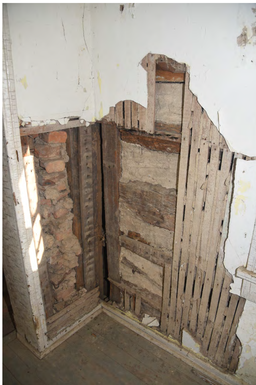
MD_FrederickCounty_Beatty-Kramer_0021.tif West room, southeast corner showing log wall with corner post.
