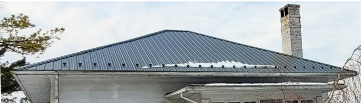
This modern metal roof has crimped, narrow panels and does not match the detailing found on an historic metal roof.
