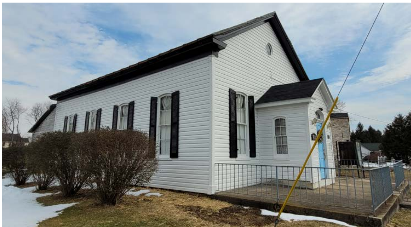
The Rocky Springs Chapel near Frederick has wood novelty drop siding.
