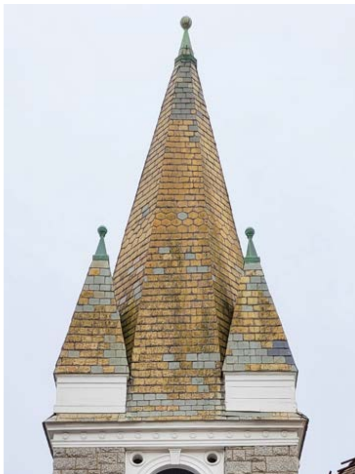
The belltower of the Buckeystown United Methodist Church is topped with a unique five pointed slate spire. The large central spire is hexagonal and the four corner spires are pyramidal. Each is topped with a finial.
