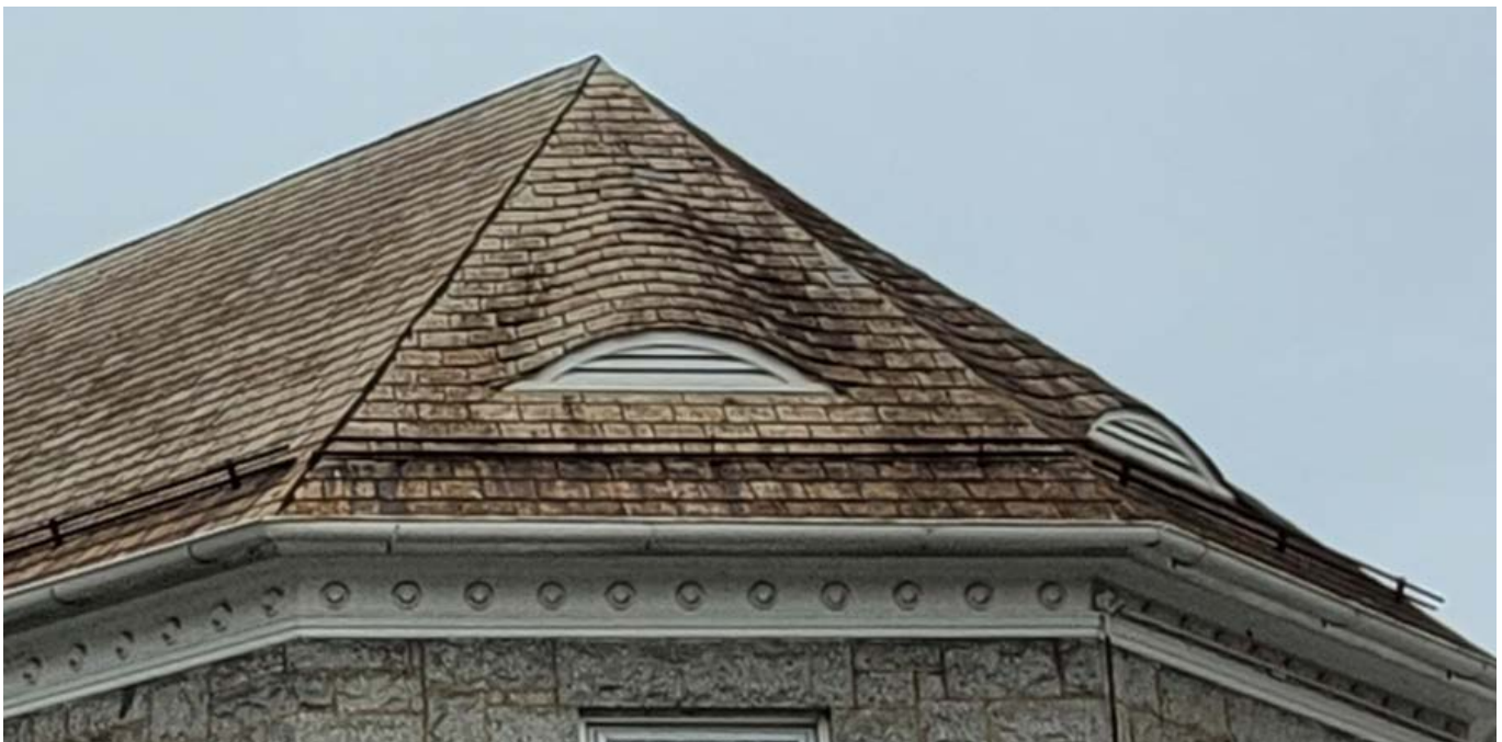
The louvers to vent the roof of Buckeystown United Methodist Church are set in small brow dormers.
