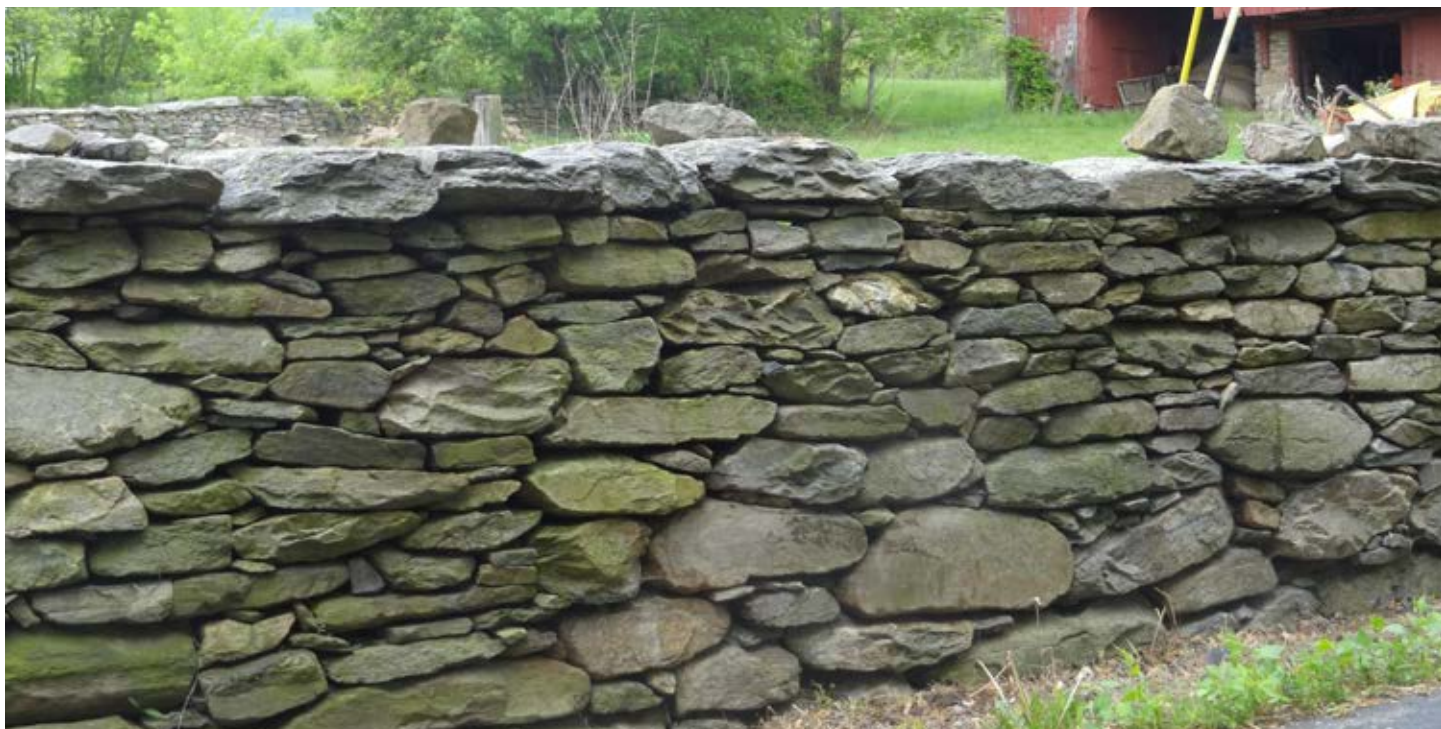
Coursed local stone wall in Burkittsville. Image Courtesy of Gary D. Baker, RA.
