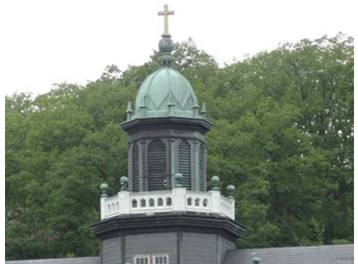
Copper-clad cupola at Mount Saint Mary's Seminary in Emmitsburg. Image courtesy of Gary D. Baker, RA.
