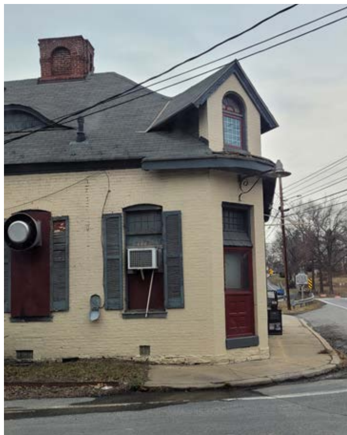
It is not recommended to modify window openings to accommodate the installation of equipment, particularly on a highly visible facade.
