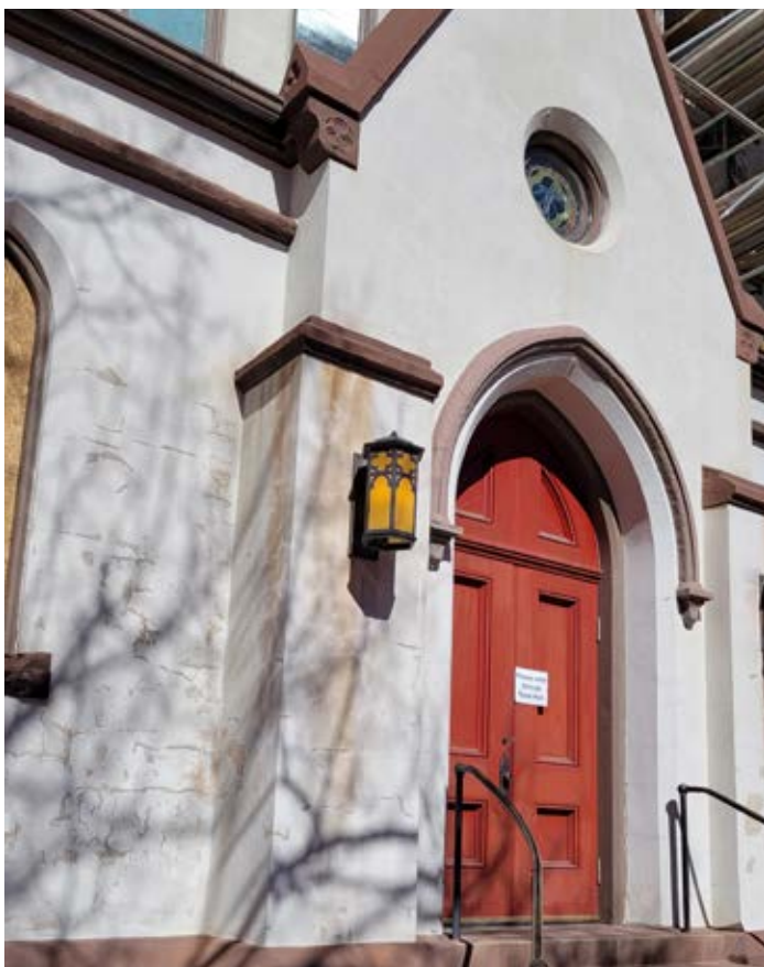
The Evangelical Lutheran Church in Frederick is made of brick walls that are covered in stucco.
