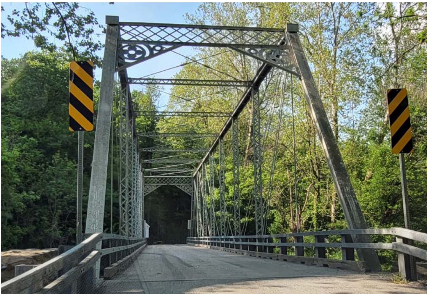
The Poffenberger Road Bridge near Middletown is an example of a Whipple thru truss iron bridge.
