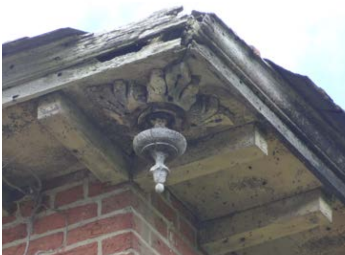
Deteriorating wooden pendant at the Point of Rocks Train Station. Image courtesy of Gary D. Baker, RA.
