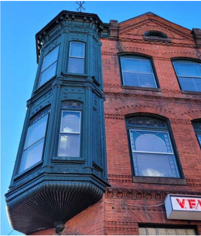
The storm windows on this building in Emmitsburg have narrow frames and align with the meeting rails of the windows, but they should be painted a dark color to match the window frames.
