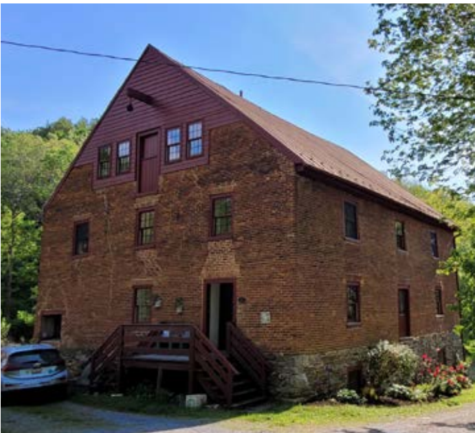
Common bond brick of the Lewis Mill in Jefferson.
