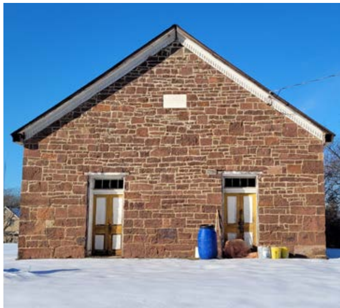
The Union Bethel Church in Creagerstown is made of stone laid in an ashlar pattern; larger stones were used for corner quoining.
