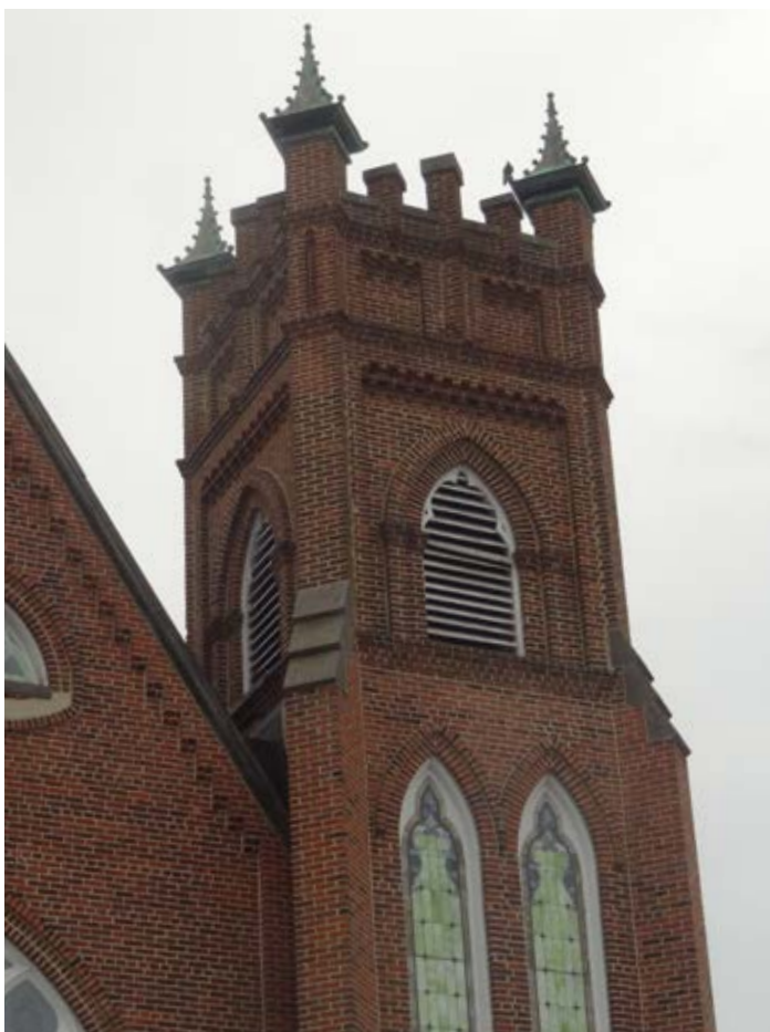
This church belltower in Emmitsburg is topped with four small copper steeple finials. Image courtesy of Gary D. Baker, RA.
