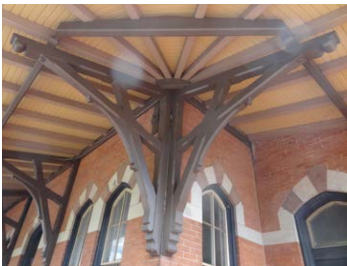
Point of Rocks Railroad Station structural framework supporting ceiling of protective overhang. Image courtesy of Gary D. Baker, RA.
