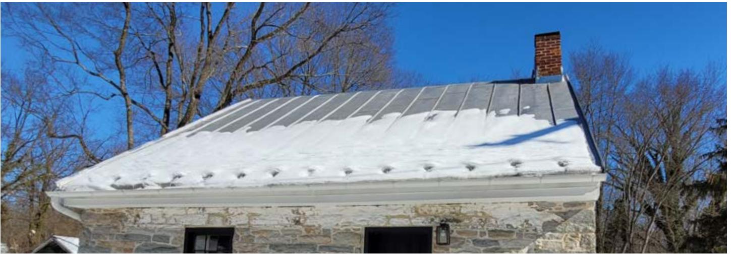
Standing seam metal roof of the Forgerman's House in Catoclin Furnace; notice the spacing of the seams and profile of the panels.
