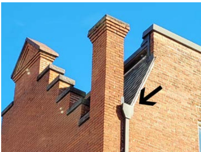
The gutters are concealed behind the brick parapet of the Sovran Bank Building in Thurmont.
