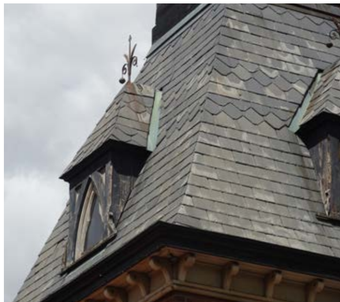
The slate roof at the Point of Rocks Train Station has dormer windows topped with finials. Image courtesy of Gary D. Baker, RA.
