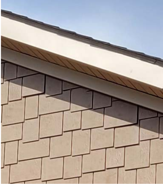
Example of a synthetic material (left) that is not an acceptable alternative for the traditional material. The synthetic shingles are too thin and flat to achieve the same profile and depth of the original.
