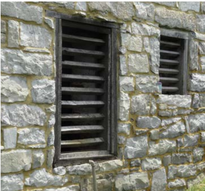
Wood louvers in a stone bank barn in Frederick County. Image courtesy of Gary D. Baker, RA.
