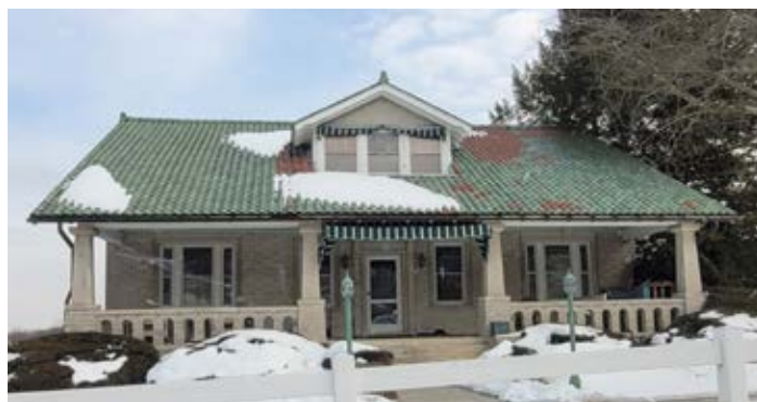
Clay tile roofing is not used frequently in Frederick County, but is seen here on this house in Braddock Heights Historic District.
