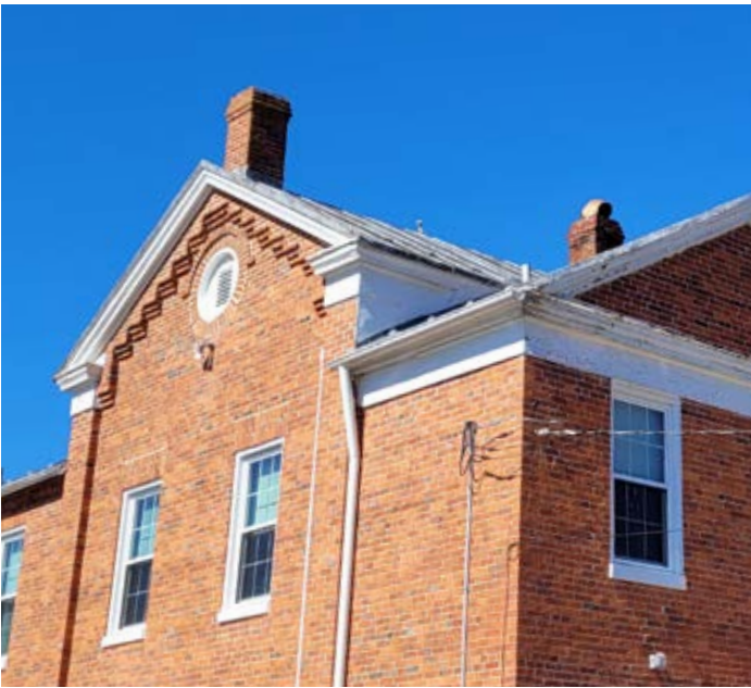
This church building in Libertytown has brick laid in Common Bond and corbelled brick at the cornice line of the gable.
