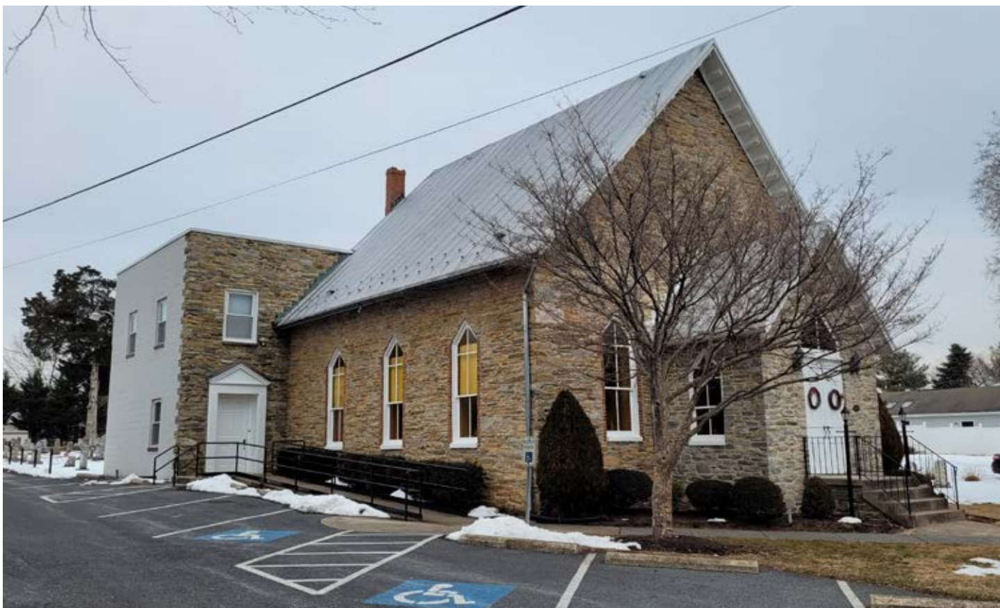
An accessible ramp and entry door was added to the Methodist Episcopal Church in Jefferson at the modern flat-roofed addition on the west side in order to keep the historic fabric of the original church entrance intact.
