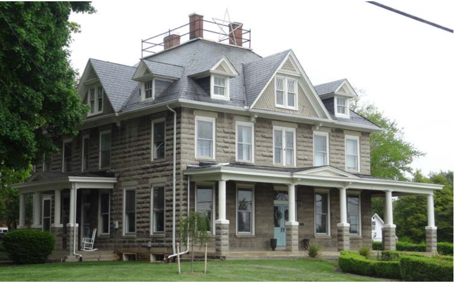
This house in Frederick County has rusticated concrete block walls. Image courtesy of Gary D. Baker, RA.
