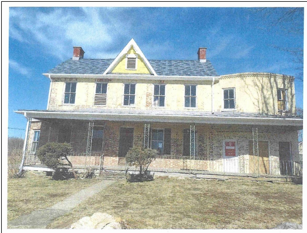
South (Façade) Elevation: Scrap & paint all openings; replace a few panes in window and French door; repair shutters.
