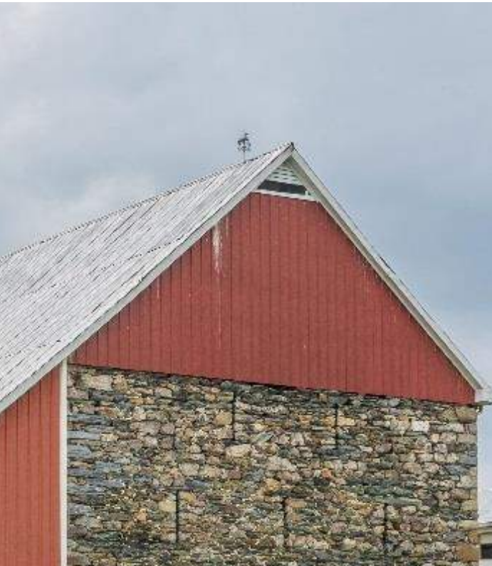
Gable ventilator near the roof of the bank barn at the Daniel James Farm. Photo by Wilson Coudon.
