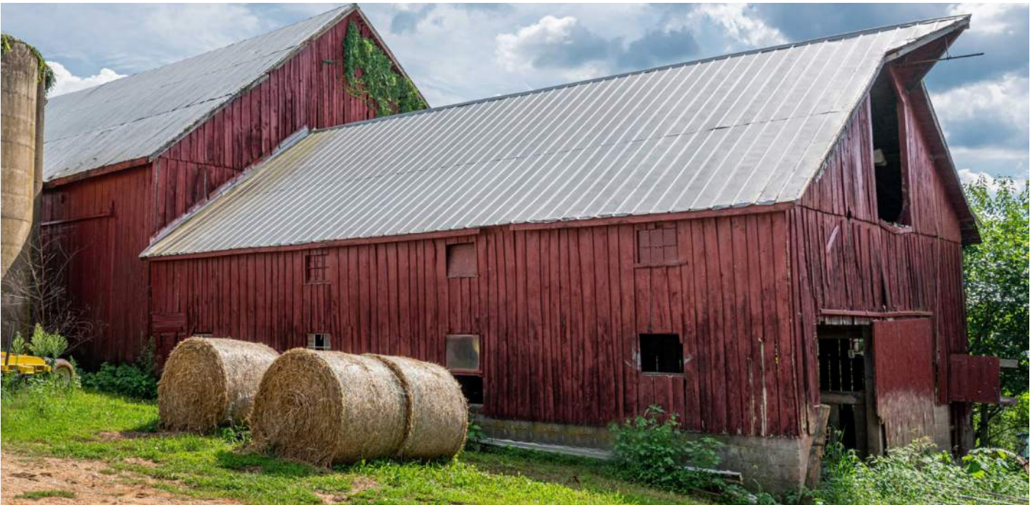
Most of the wood siding found in Peace and Plenty is vertical board-and-battens like that of the bank barn at the William Downey farm. Photo by Wilson Coudon.
