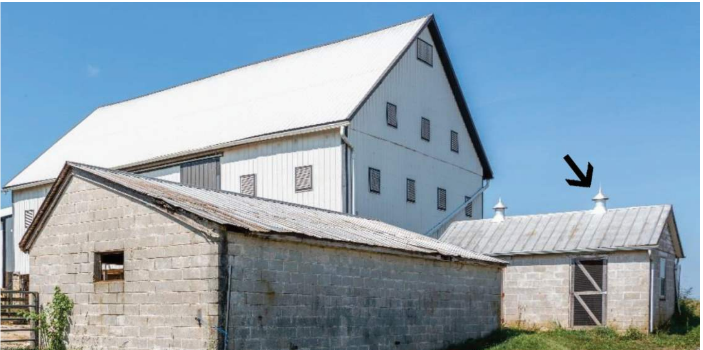
The bank barn at the Captain Ignatius W. Dorsey Farm has been resided in metal and the adjoining milk house has distinctive “oil can” shaped metal vents. Photo by Wilson Coudon.
