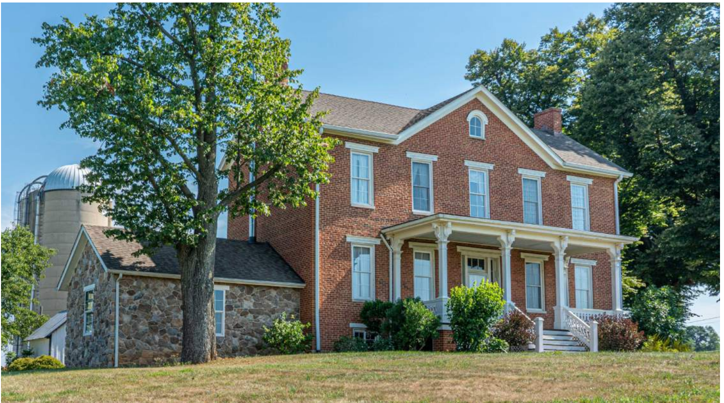
The brick of the Captain Ignatius W. Dorsey farmhouse is laid in a common bond pattern. Photo by Wilson Coudon.
