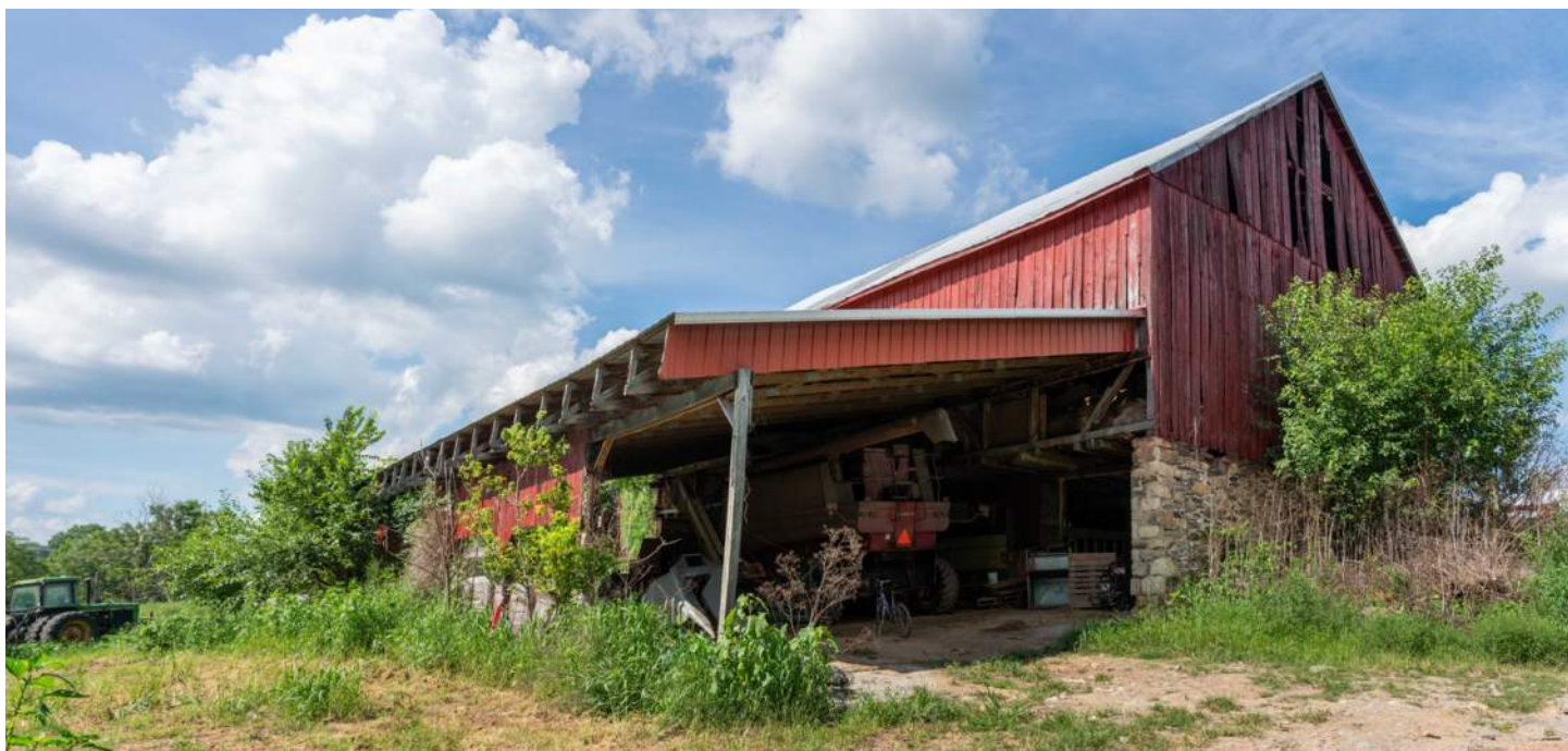
Simple barn forms with gable roofs were often expanded with shorter shed structures like this bank barn at the Wright Downey Farmstead. Photo by Wilson Coudon.
