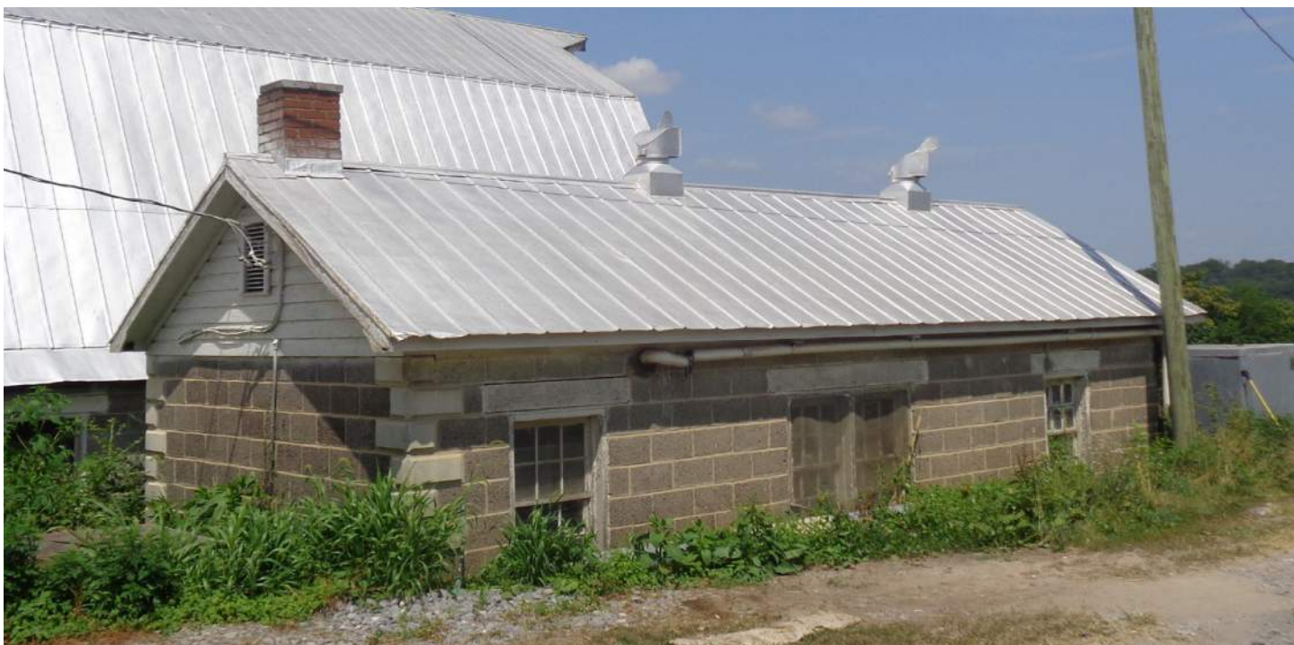
The milk house at the Wright Downey Farmstead has walls made of concrete masonry units. Photo by authors.
