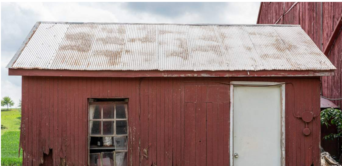
Corrugated metal roofing on this small ancillary structure. Photo by Wilson Coudon.
