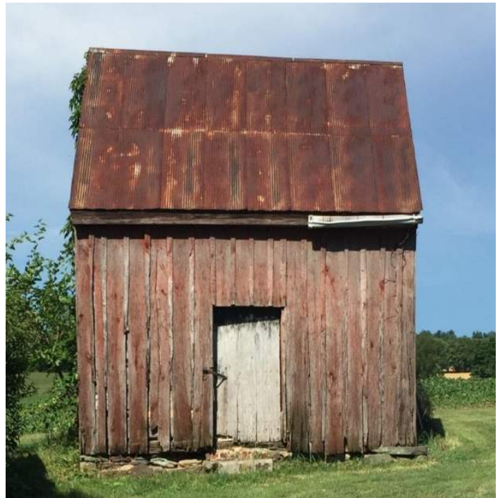
This smoke house on the William Downey farm is a log structure with wood siding. Photo by Wilson Coudon.
