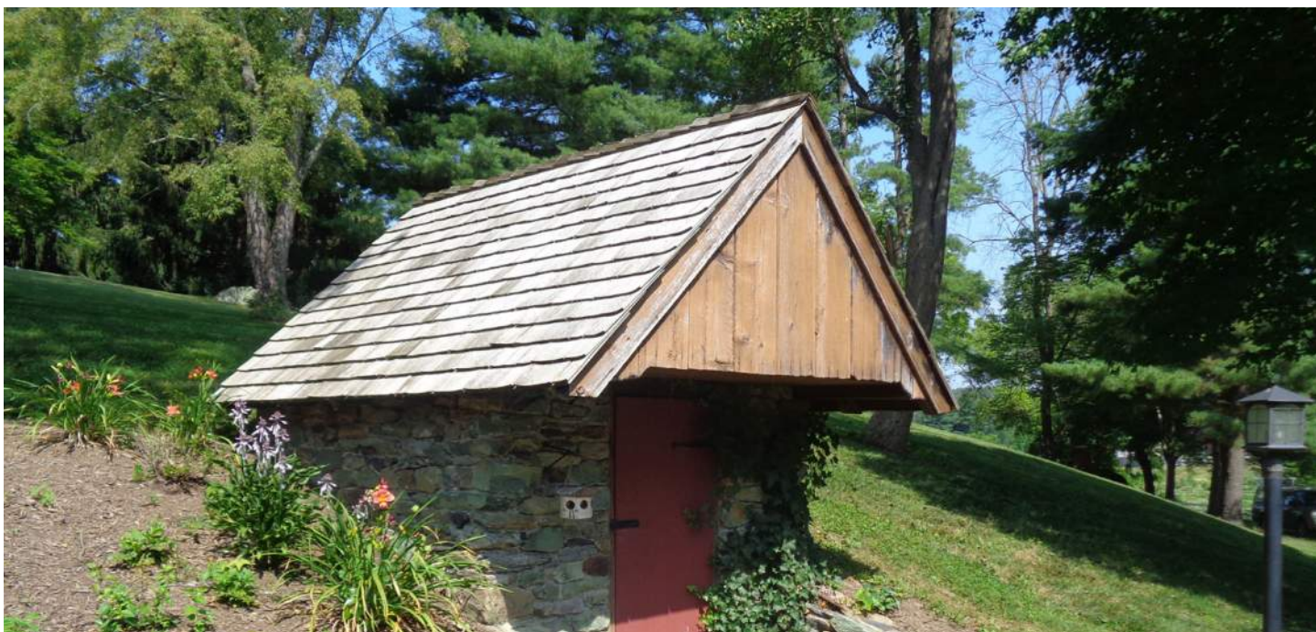
Wood shingle roofing on an ancillary structure at Still Work Farm. Photo by authors.
