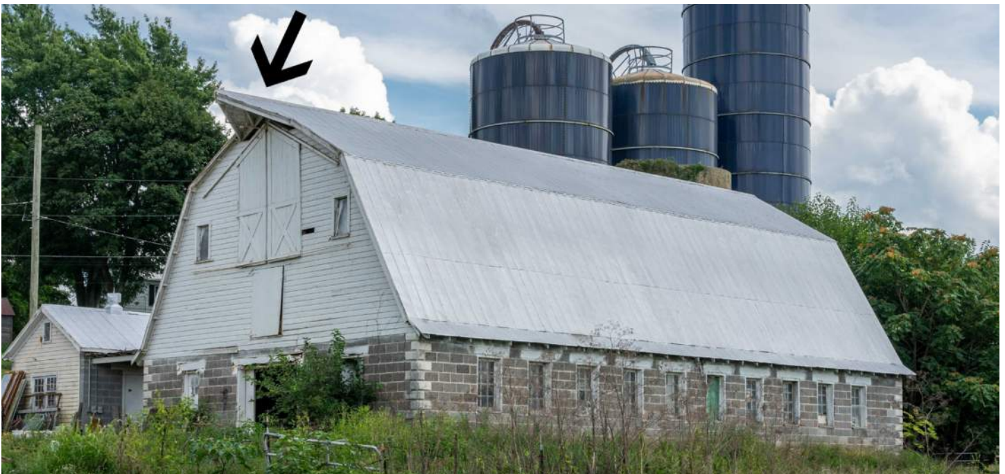
The dairy barn at the Wright Downey Farmstead has a prominent gambrel roof form with a hay hood at the end of the ridge. Photo by Wilson Coudon.
