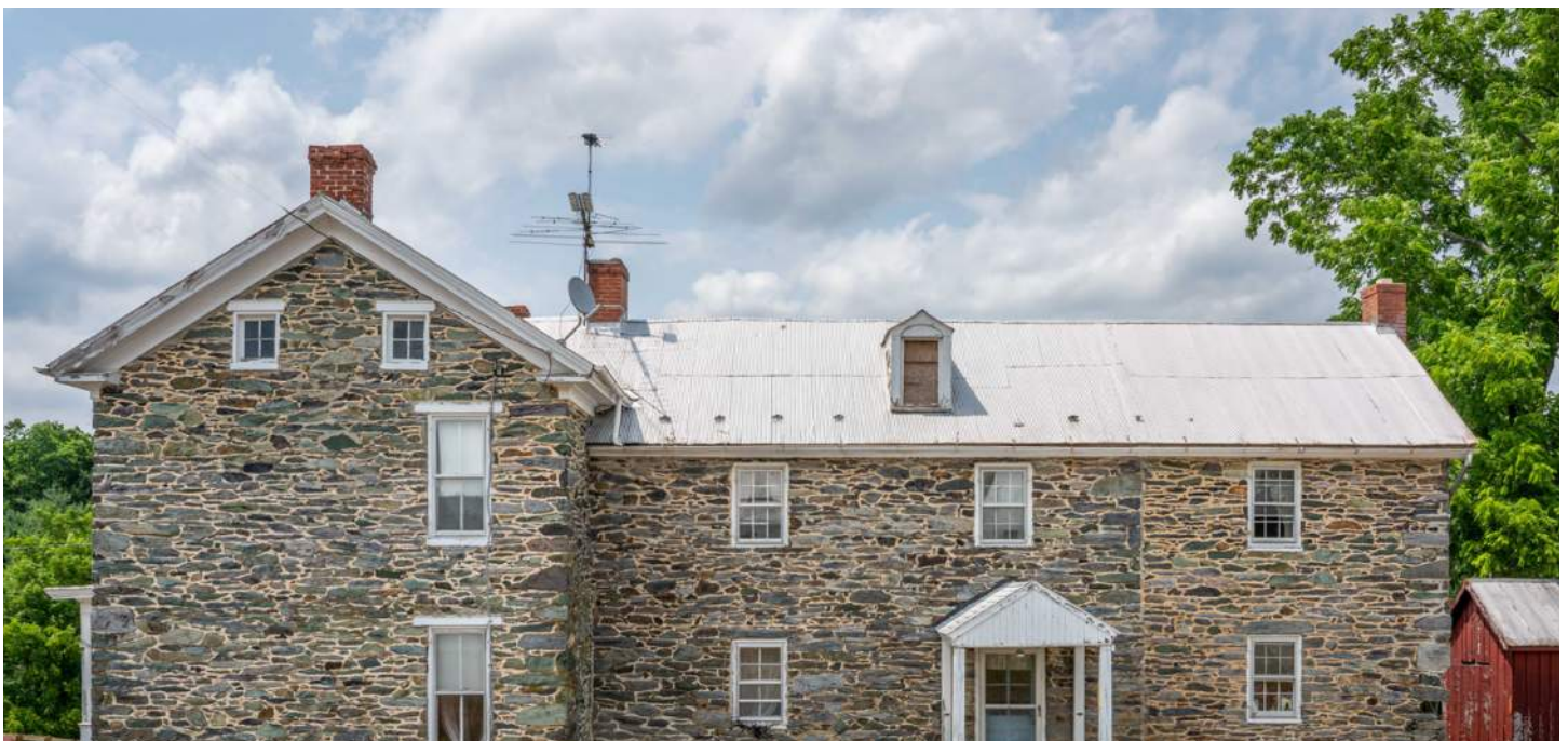
Sheet metal roofing on the Basil Harding farmhouse. Photo by Wilson Coudon.
