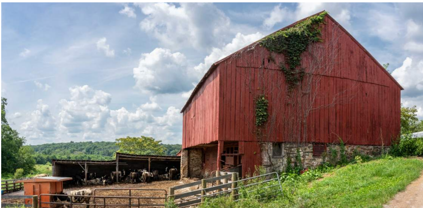
The upper structure of the bank barn at the Wright Downey Farmstead was rebuilt upon its stone foundation walls. Photo by Wilson Coudon.
