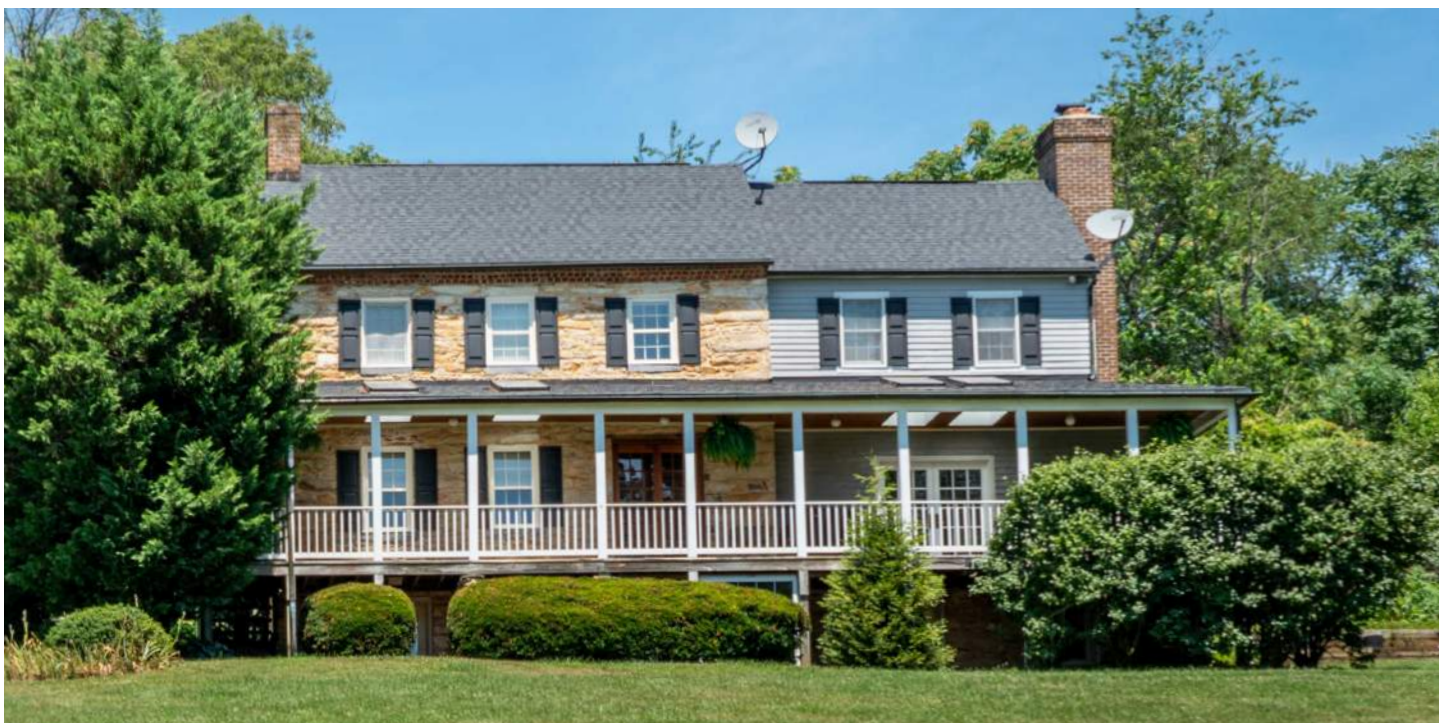
The rear elevation of the Vernon Dorsey House has a porch that extends across the width of the building linking the early stone structure with the newer frame addition. Photo by Wilson Coudon.
