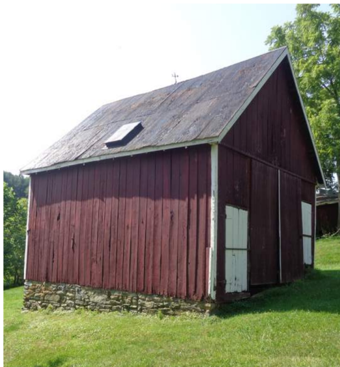
This ancillary structure at Still Work has vertical board siding. Photo by authors.
