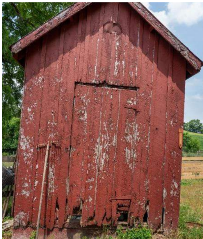
Board-and-batten door at the smokehouse at the Basil Harding Farm matches the siding. Photo by Wilson Coudon.
