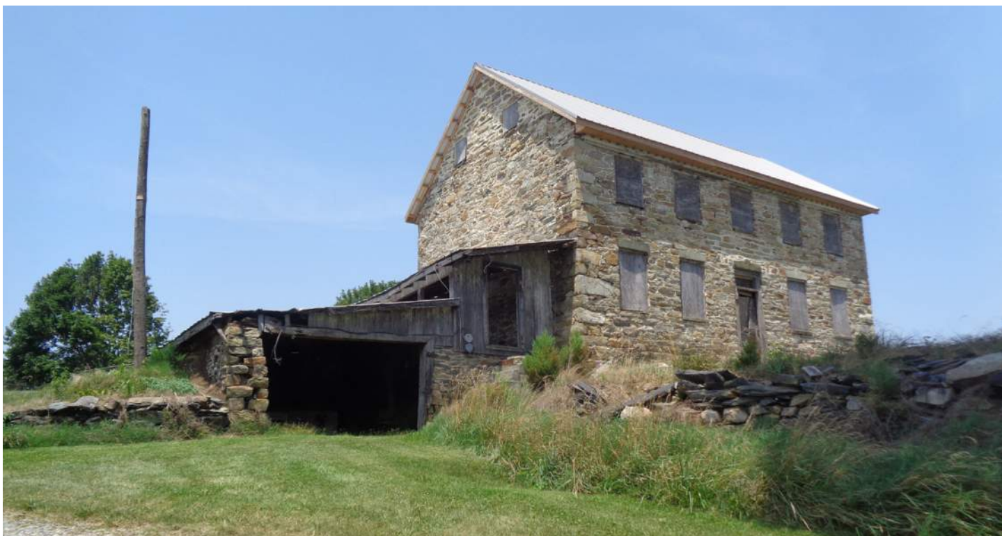
Stone retaining walls extend beyond the walls of the Daniel James house. Photo by authors.
