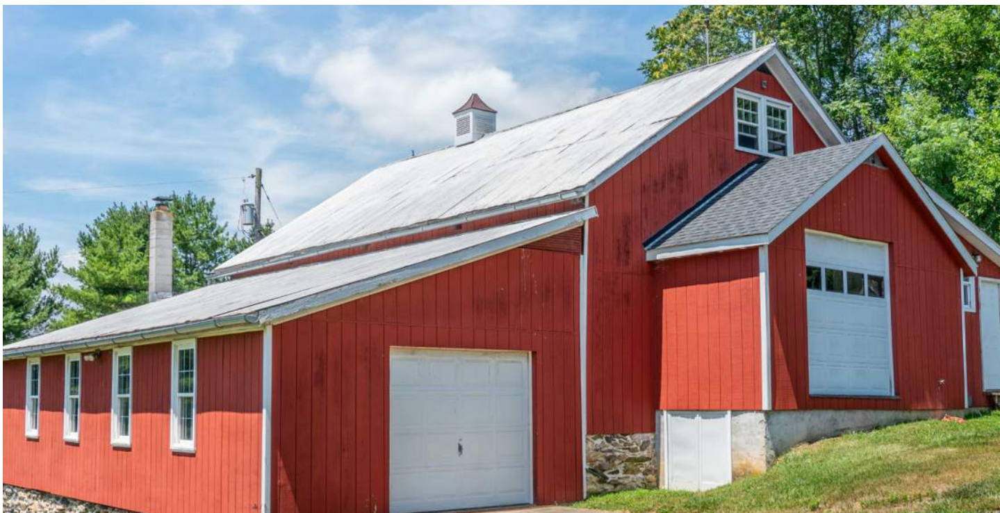
Plywood siding board is an alternative material found on this newer agricultural building at the Samuel Dorsey Farm. Photo by Wilson Coudon.
