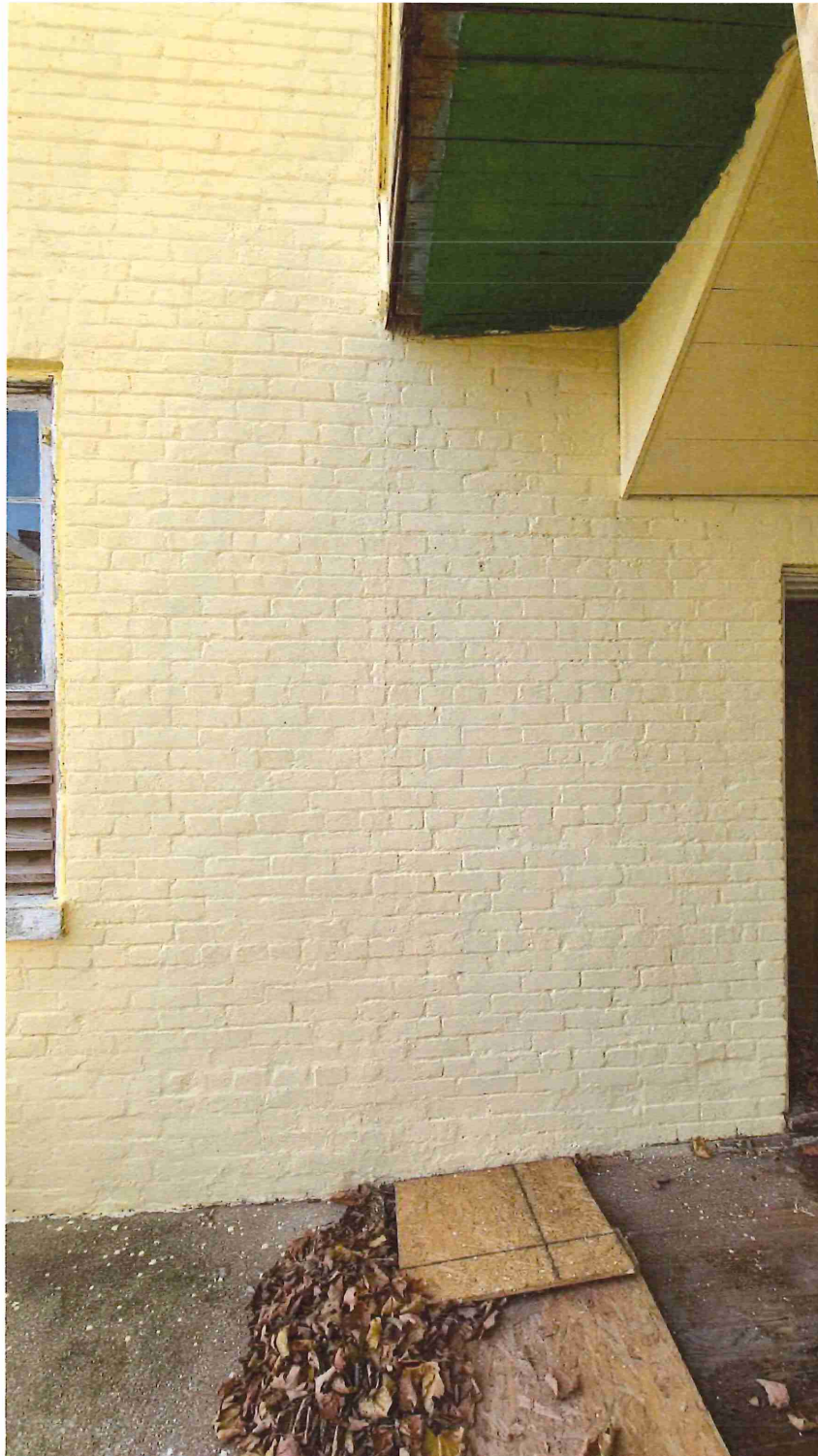
Photograph 3: Exterior common bond brick wall along the south side of the porch. Note how there are no signs of attachment between the removed wall and the brick wall. Also the paint change on the ceiling is visible.
