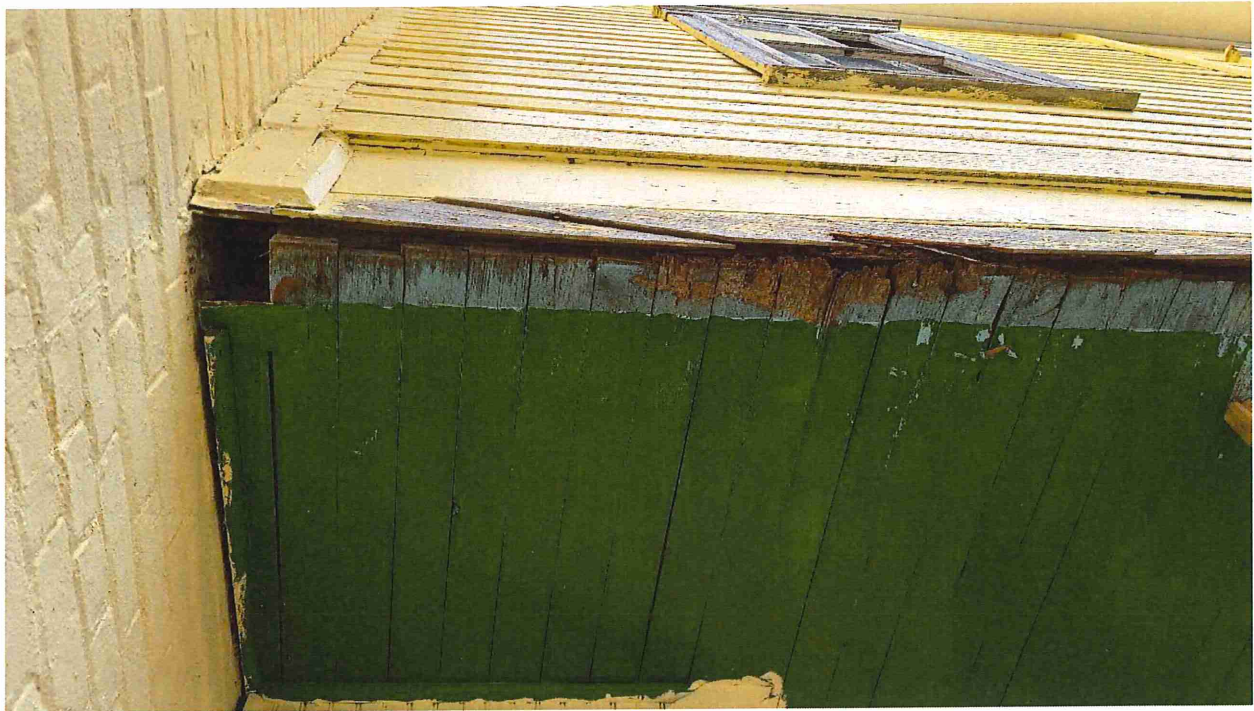
Photograph 4: Paint found on the porch ceiling under the wall that enclosed the porch. The color closely matches the painted front porch.
