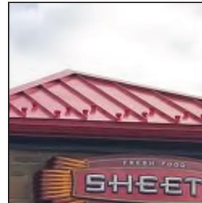
(10): STANDING SEAM METAL ROOF MFR: PAC-CLAD PETERSON, A CARLISLE COMPANY FIN: CARDINAL RED
