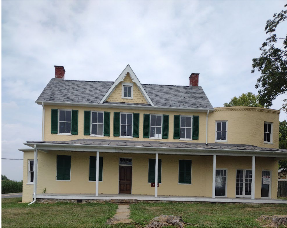
Image 3: Front porch with wooden columns and iron elements removed
