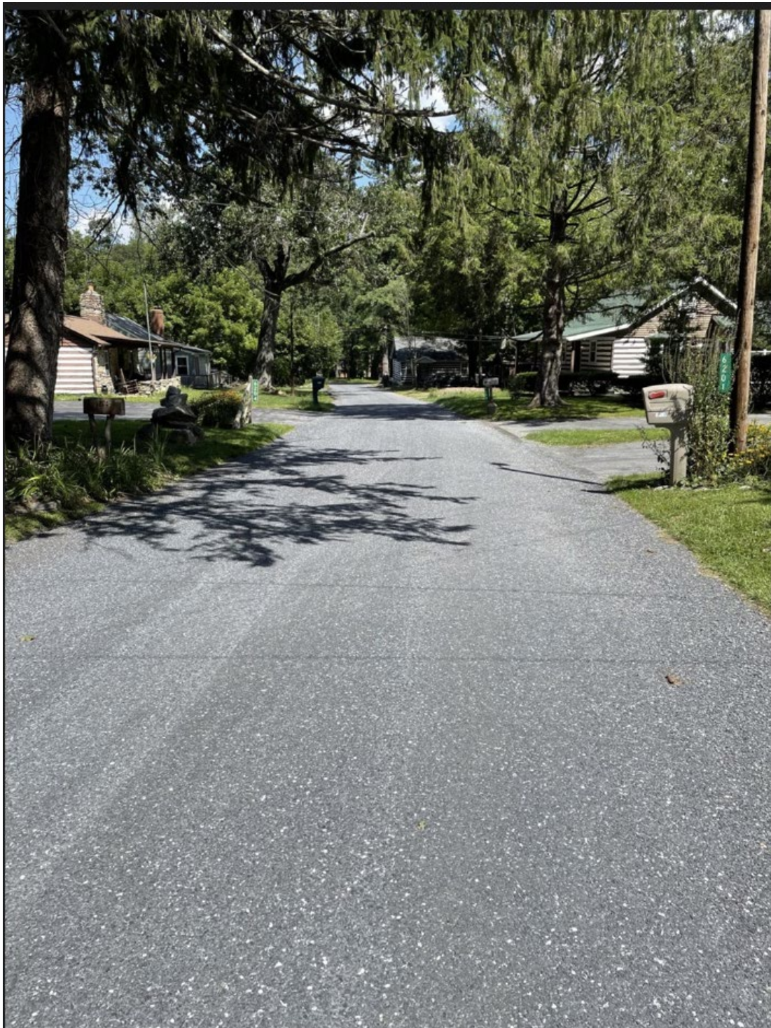
Figure 1.2: New tar and chip treatment with no fog seal. Mountaindale Road applied 7/1/2025
