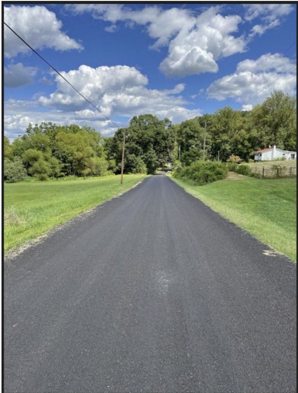
Figure 1.1: New fog seal treatment on Links Bridge Lane applied 7/21/2025.
