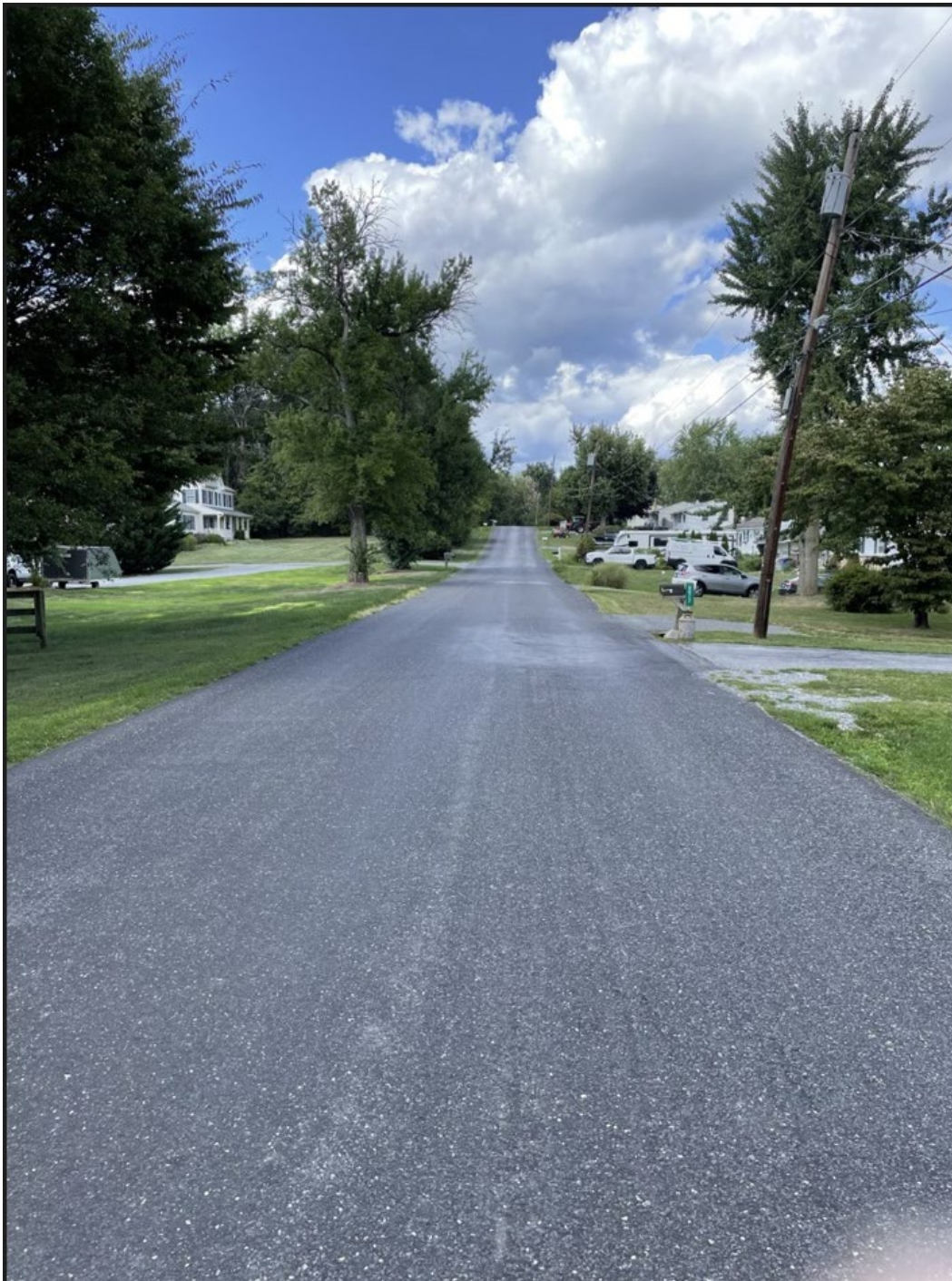
Figure 2.2: Chestnut Grove Road fog sealed on 10/19/2023.
