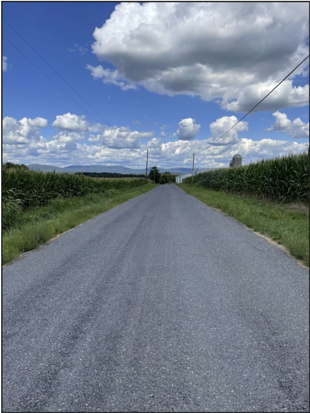
Figure 3.3: Wilhide Road just off of Lewistown Road. Tar and chip no fog seal applied on 9/20/2021. Signs of bleeding.
