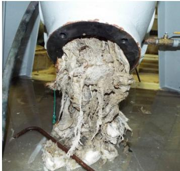
Here is something to consider: This is an image from a clogged pump in a Frederick County sewage pumping station caused by 'flushable' wipes. If they are able to completely block a pump in a high capacity sewage pumping station, just imagine what could happen inside of your own home or business that has much smaller sewer lines?
