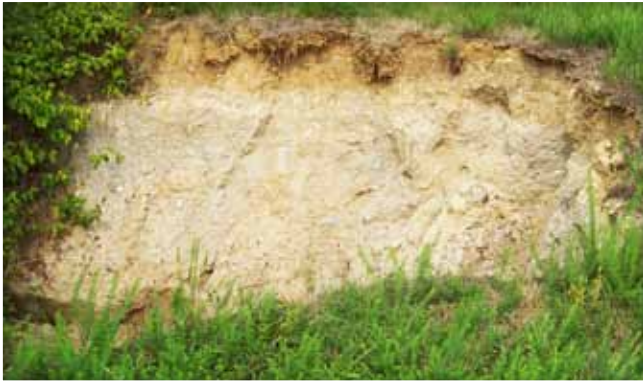
Slope erosion or failure on dam (embankment).
