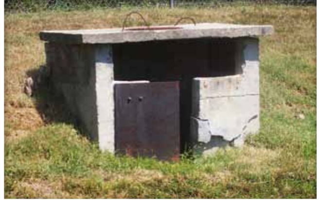
Broken or damaged control structure.
