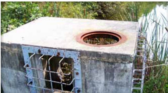
Missing manhole cover on control structure.
