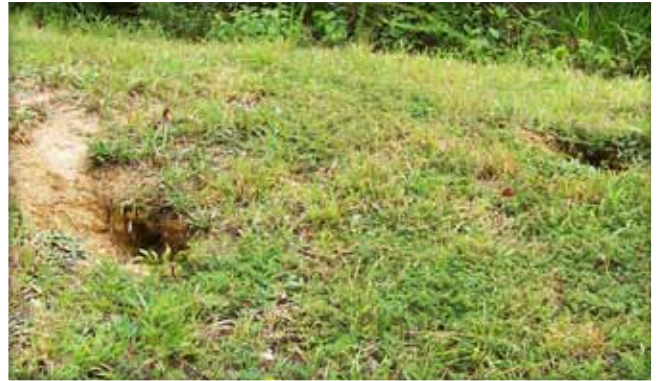
Animal burrows in the dam embankment; beaver lodges blocking outlet pipes.
