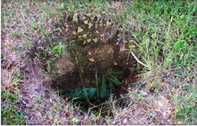
Cracks or sink holes on dam (embankment).
