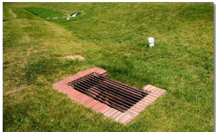
Bioswale along Needwood Road Bike Path / Trail source: JMT
