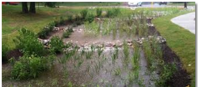
Submerged Gravel Wetland source: Montgomery County
