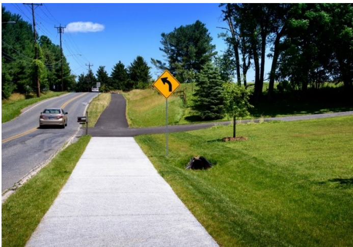
Permeable Pavement along Needwood Road source: JMT
