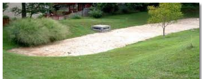
Surface Sand Filter source: Montgomery County
