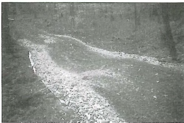
Wet area in road being stabilized with geotextile and stone.
