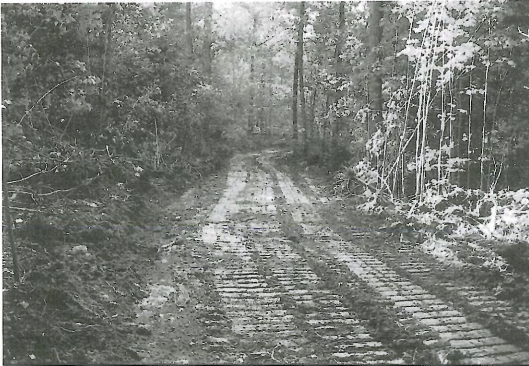
Newly constructed truck haul road with 2% grade.
