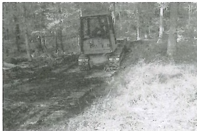
Broad-based dip being constructed on truck haul road.
