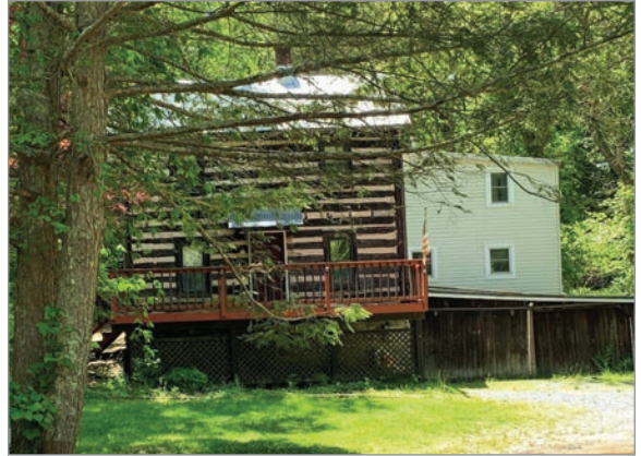
The Abraham R. Simmons House, located off of Thurston Road, is a two-story log dwelling with a modern addition. The house was probably built circa 1850 in the vicinity of a mill known as Simmons Mill (now demolished) on Bennett Creek. The house likely had a two-story porch on the façade, which has been replaced with a deck. The Maryland Historical Trust records identify this historic resource as MIHP F-7-72.
