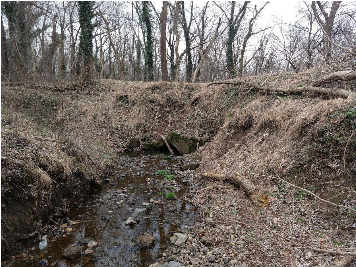
Figure 3. The largely buried culvert under the C&O canal downstream of the project
