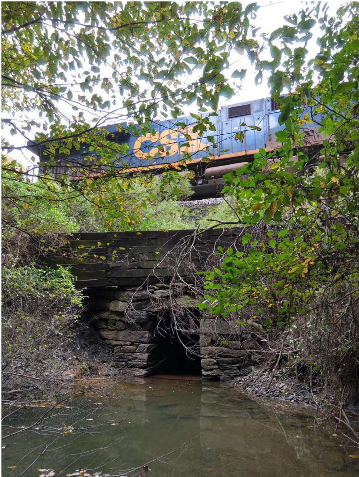
Figure 5. MD-28 culvert - legacy 4 ft x 5 ft box culvert under CSX tracks (outflow/downstream face)
