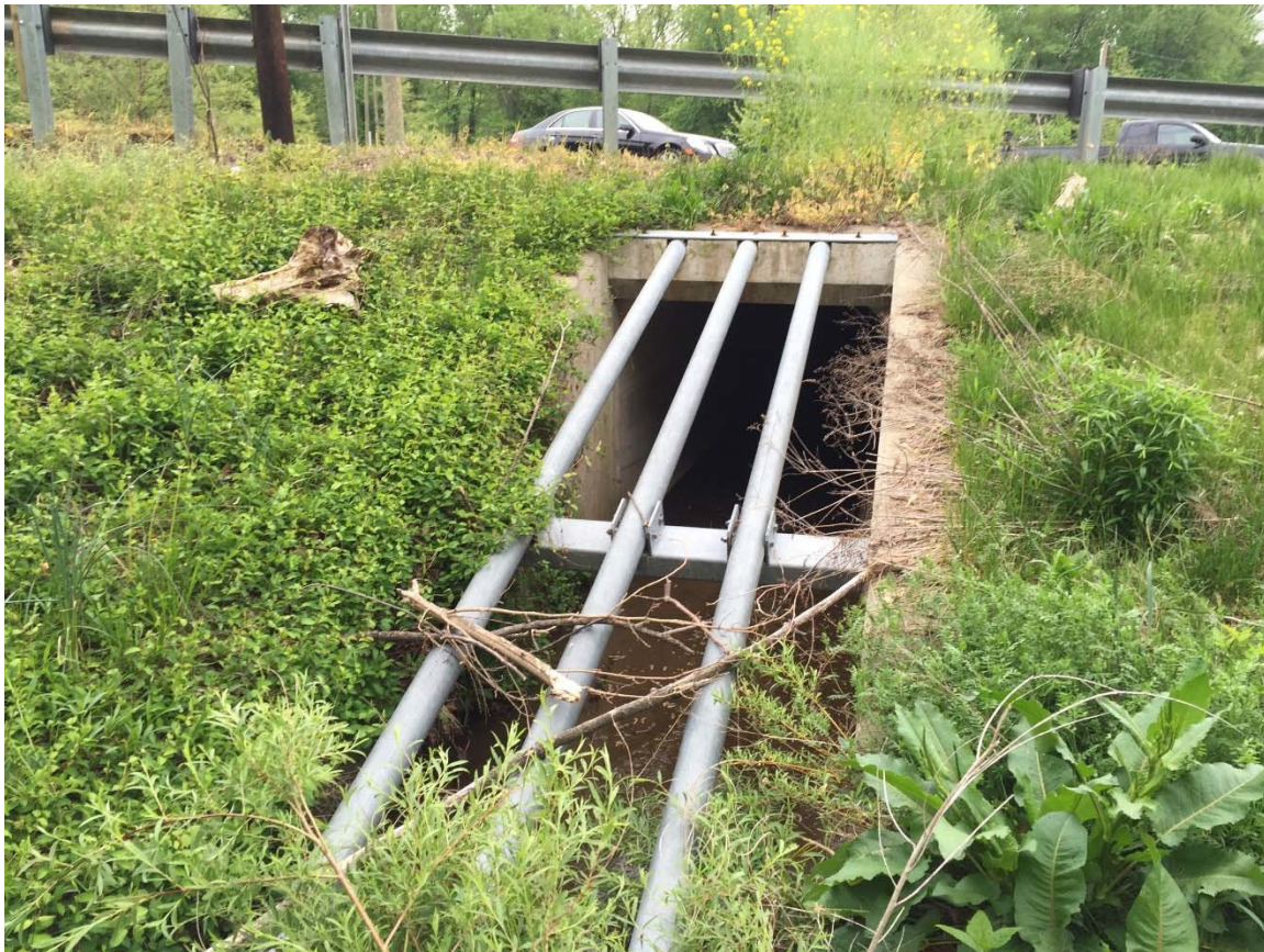
Figure 6. MD-28 culvert - 5.5 ft x 5.0 ft box culvert inflow/upstream face
