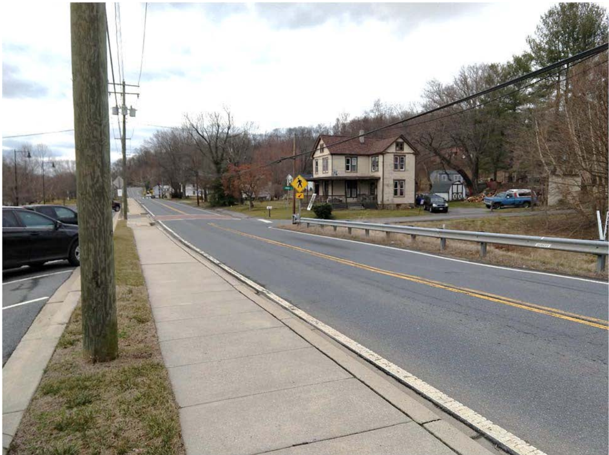
Figure 9. Downstream flood hazard areas. MD-28 and its sidewalk are in the center. The brown house on the right is 3744 Clay Street. The MDOT MTA parking lot is on the left, separated from the sidewalk by a grass strip
