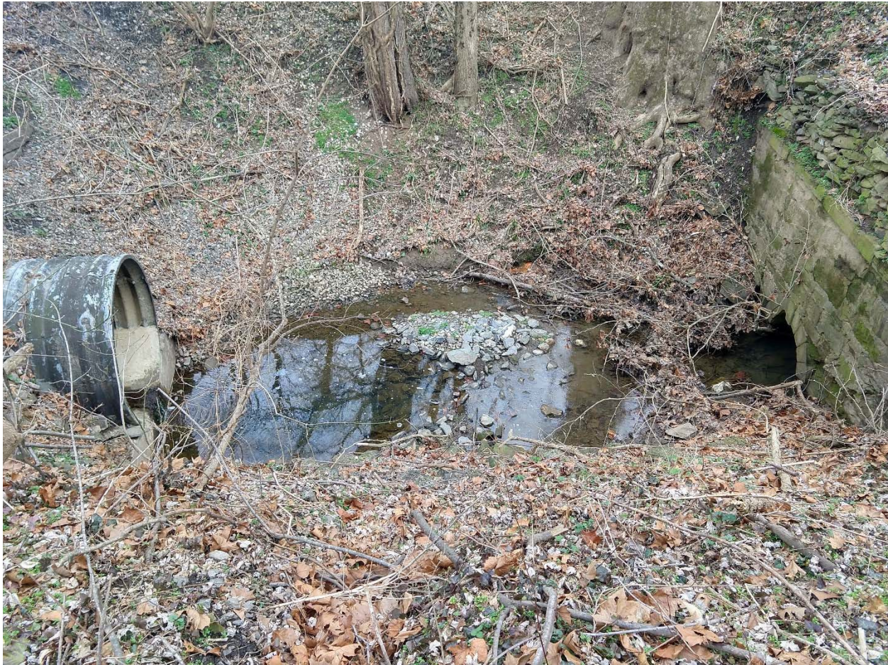
Figure 4. The western boundary between the CSX railroad (CMP culvert on the left) and the C&O canal (stone culvert on the right)
