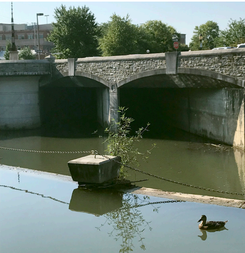
Culverts of Frederick's Carroll Creek flood control project
