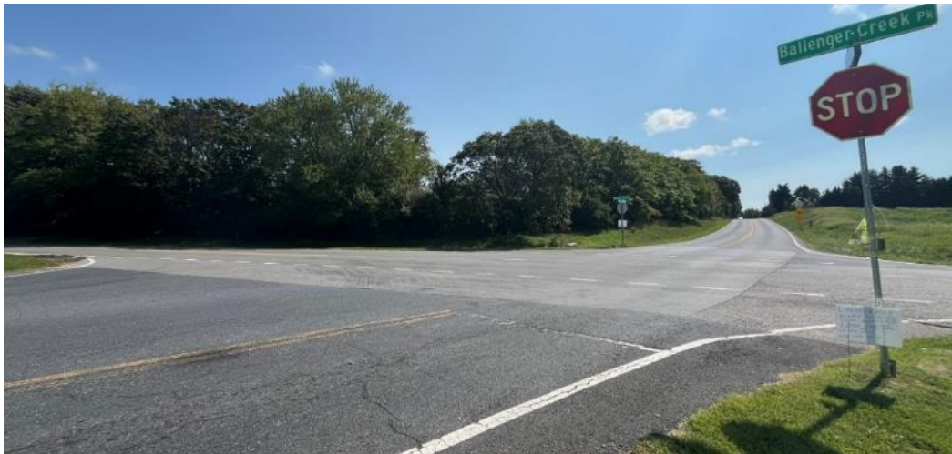
Figure 24: Faded pavement marking/stop bar at Mountville Road and Ballenger Creek Pike
