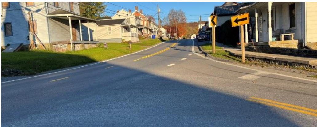
Figure 10: Poorly visible pavement markings (Sabillasville Road and Harbaugh Valley Road Intersection)
