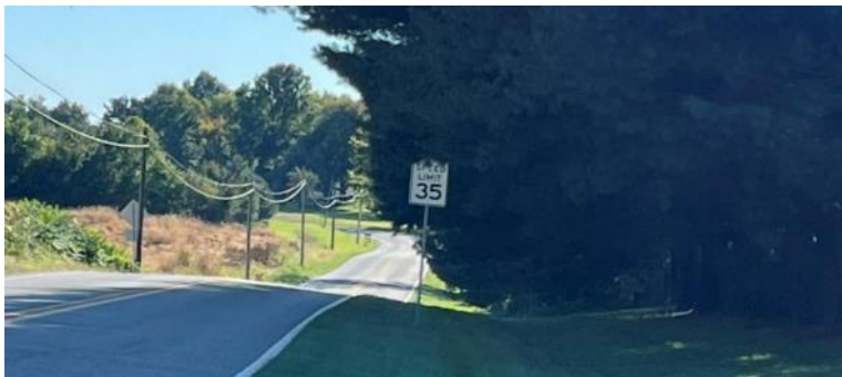
Figure 25: Obstructed speed limit sign along westbound Ballenger Creek near Mountville Road
