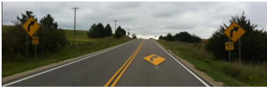
Figure 30: Sample Curve Sign pavement marking from Lecompton, KS (FHWA Traffic Control Devices Pooled Fund Study: Evaluation of Elongated Pavement Marking Signs, October 2014)
