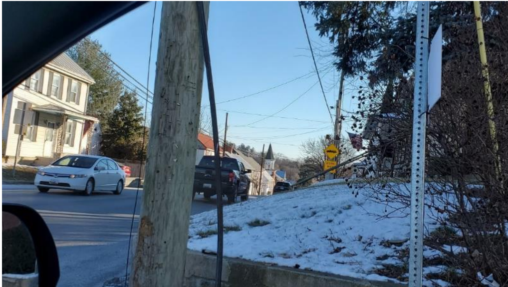
Figure 5: NB Mill Street at MD 26 – looking right (Note: utility pole, shrubbery and topography restricting available sight distance)
