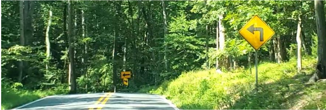
Figure 29: Southbound Dance Hall Road approaching sharp turn – Note: Turn (W1-1) sign is faded and dirty
