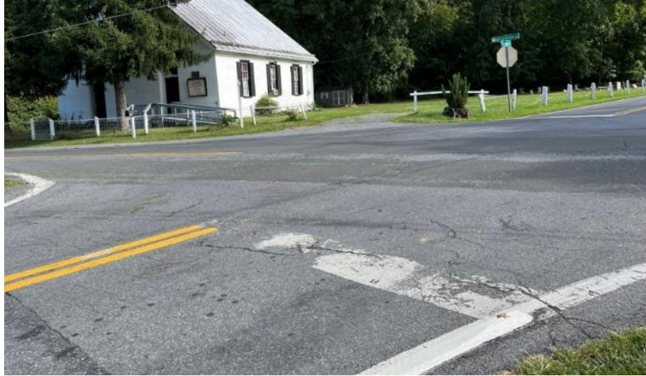
Figure 21: Faded Markings at Mountaindale Road and Bethel Road Intersection
